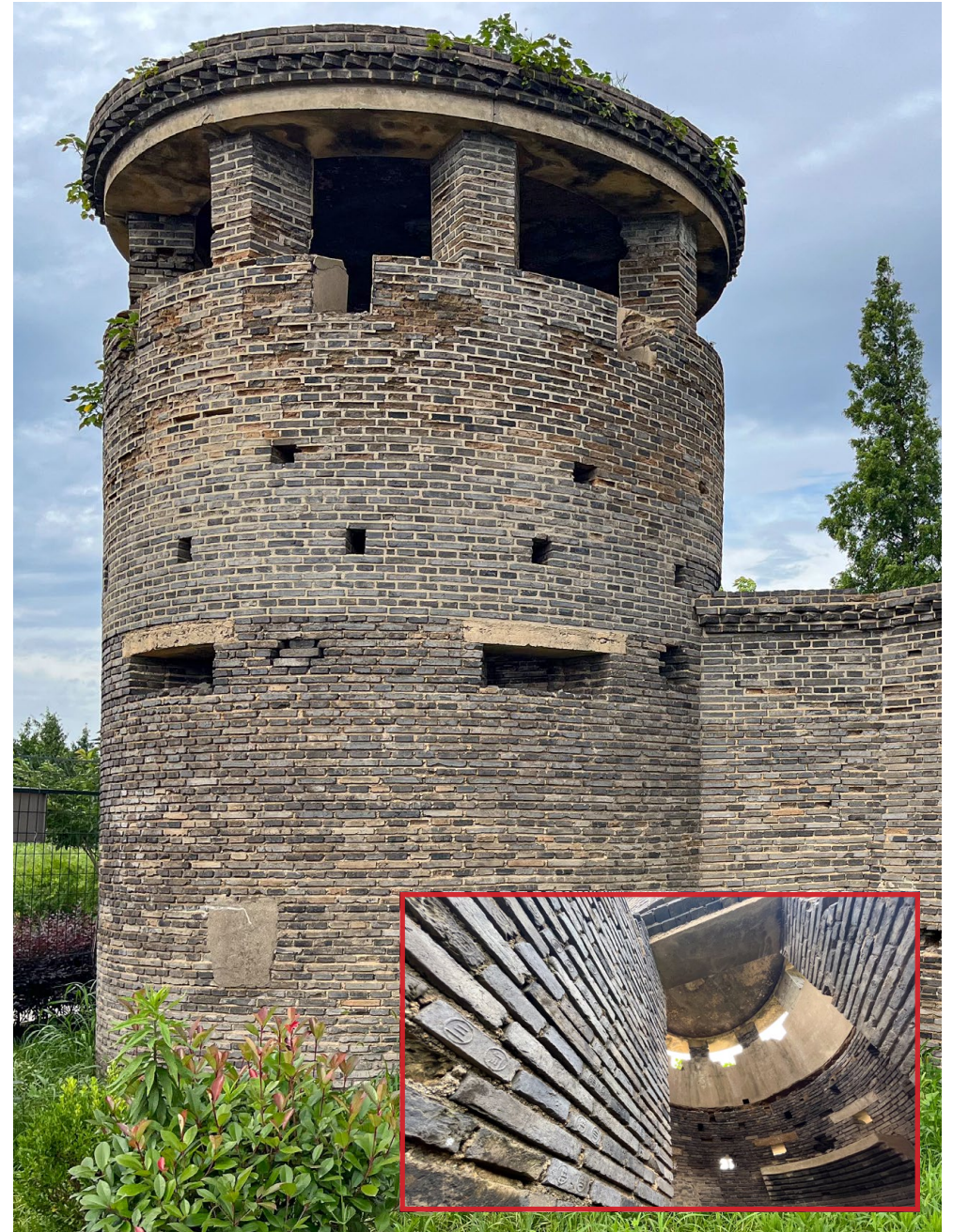
Xinbang Fort, a Japanese masonry blockhouse at a former railway river crossing in Songjiang district. The small holes are not loopholes, but were to uphold the supports for a wooden floor. Inset shows interior.
