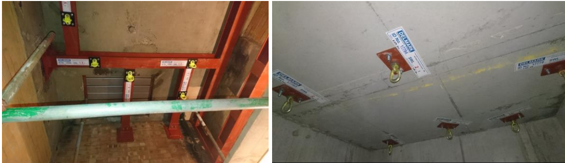
Figure 1: Steel Lift Shaft Beam with lifting eyes (left) and Concrete slab with lifting eyes (right).
