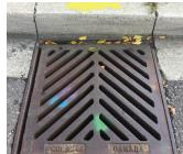
Lake Ontario. Our stormwater drainage system helps to make sure that water flows away from roads and properties to reduce the risk of flooding, damage, erosion or wet areas. Keep catchbasins near your driveway or in your backyard
