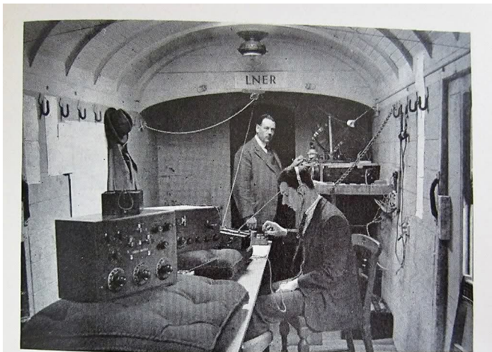
Radio coach 6ZZ left King's Cross station on July 5, 1924, attached to the 7.38 p.m. Scottish express of the (then) London and North Eastern Railway. The occasion was an experiment carried out by members of the Radio Society of Great Britain to test the practicability of maintaining radio communication between a train travelling at high speed and fixed stations along the route using amateur equipment. In this picture Maurice Child is at the key and Leslie McMichael is adjusting the transmitter which operated on 182.5 metres. Two-way contact was established with 2WD (Bedford), 5DR (Sheffield), 2DR (Shipley) and 5MO (Newcastle-on-Tyne).
