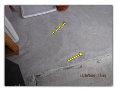
FYI: One or more hairline cracks were observed at the foundation grade beam surfaces (South). These cracks, by themselves, do not necessarily indicate the presence of serious structural issues with the foundation, and are typically localized in the cosmetic parge coat applied to the surface of the grade beam. However, any cracks observed at the foundation grade beams should be monitored for future movement or increase in size over time.
