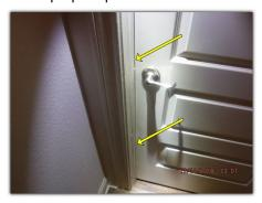
**Poor seal observed at door weatherstripping** (*front entry door*). Weatherstripping improvement is recommended where necessary in order to prevent possible water and / or insect penetration and air drafts around the perimeter of the door(s).
