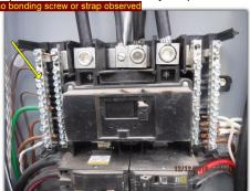
**Paint / texture over spray observed inside panel box** (garage panel). All internal parts of any panel box (bus bars, wiring terminals, insulators, etc.) are not to be contaminated by foreign materials (paints, plasters, cleaners, etc.). It is recommended that you consult with a licensed electrician or the panel box manufacturer in order to determine how to properly address the over spray as some of the over spray was also observed on the live bus bars.
