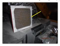
(manual fixed damper observed, but no timed or Suspected incomplete installation of fresh air return system automated damper system). An HVAC system with a constant and continuous supply of outdoor air may not operate efficiently and may have trouble regulating humidity within the home. Further evaluation and repair is recommended as required by a qualified heating and cooling technician.
