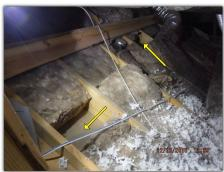
**Missing blocking at wall sheathing seams / joints** (South gable wall above front living room). All edges / seams of the exterior wall sheathing should be properly supported / blocked in order to resist movement; particularly when stucco wall coverings systems are present as movement within the sheathing can lead to stucco cracking. Monitoring and repair is recommended as necessary.
