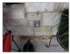
**Potentially under-sized wiring observed to be serving condenser unit** (suspected 30 amp wiring on a condenser unit with 34.8 minimum ampacity rating). Further evaluation and repair is recommended by a qualified electrician for proper wiring / equipment protection.
