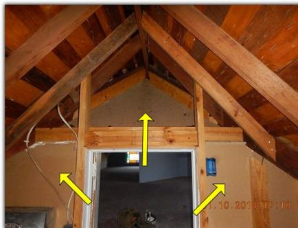
**Missing or gapped fireblocking** (*observed from attic, near the front chimney structure*). Fireblocking shall be provided to cut off all concealed draft openings and to form an effective fire barrier between vertical and horizontal spaces within the structure (*in this case, between wall voids and the attic space*). These gaps / openings should be properly sealed off with solid lumber, metal or tightly packed, unfaced fiberglass insulation for improved safety.
