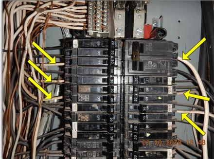
**Missing wire clamps and knockout plates.** All wiring passing through metal panel boxes shall be properly protected from abrasion damage and all openings in panel boxes or their covers should be filled with the appropriate fill plates/covers in order to prevent shock hazards and potential damage to the components inside the boxes.
