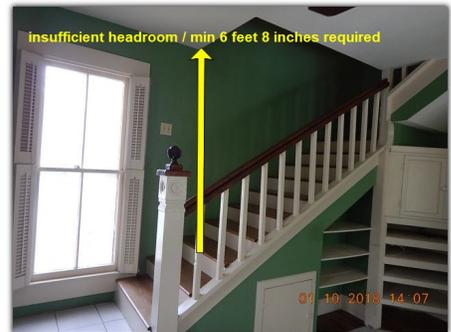
**Loose / leaning newel post and handrail (smaller stairway near North entrance).** Repairs are recommended.
