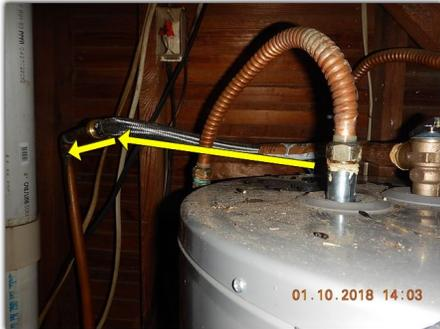
**Ungrounded electric water heater** (*upstairs unit*). Further evaluation and repairs are recommended for improved safety.
