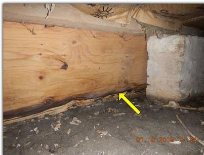
**Missing hangers and poor support at opening in floor framing** (where older in-floor furnace is located at North side of home). Although no evidence of movement or sagging was observed at this portion of the floor structure, monitoring is recommended.
