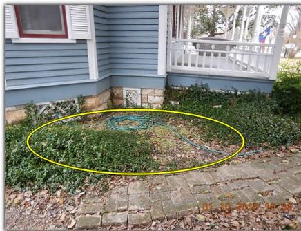
**High soil against the foundation/structure (detached garage).** Ideally, the soil line should remain 4-6 inches below the bottom edge of the siding in order to prevent possible moisture penetration or potential wood-destroying insect activity. In some cases, where correcting the high soil creates a negative grade against the foundation, underground drainage options may need to be explored.
