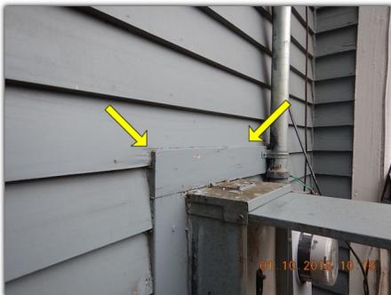
**Loose / unsecured siding observed** (multiple locations). Further evaluation and repairs are recommended where necessary.
