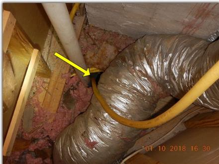
**Improperly installed insulation batts** (*various locations where combustible paper is exposed and not against drywall*). The insulation manufacturer states that the combustible paper facing should not be exposed as it is a potential burn / fire hazard (*instead should be facing drywall, insulation, etc.*). Repairs are recommended as necessary for improved safety.
