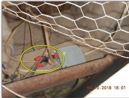
**Improper dimmer switches for ceiling fan motor use** (*middle bedroom -- front bedroom*). Some of the dimmer switches used for ceiling fan are not approved for use with a ceiling fan (*incandescent fixtures only*). This condition can be a potential fire hazard due to overheating. Proper switch replacement is recommended where required for improved safety.
