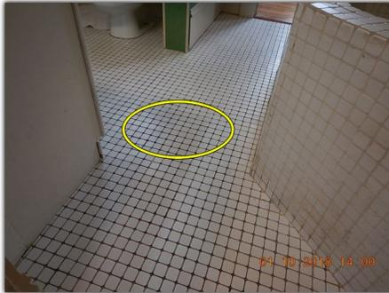
**Uneven floor surface and cracked floor tiles** (*rear bonus room off of kitchen*).
