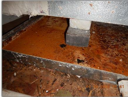
**Improper condensate drain line configuration (*upstairs unit*).** The primary and auxiliary drain lines were observed to be tied together and terminating close to the foundation. Furthermore, the evaporator coil drain pan line was observed to terminate at the rear exterior, but not directly above a window or door opening, as required. Further evaluation and repairs are recommended by a qualified heating and cooling technician.
