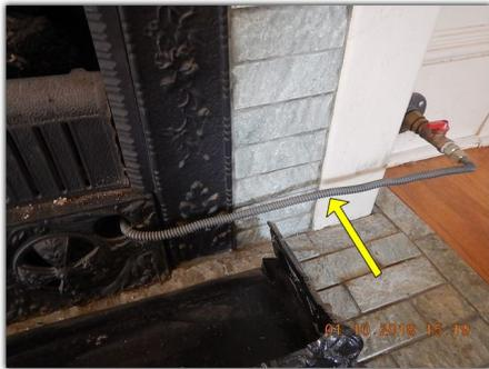
**Missing protective jacket and exposed CSST gas lines** (*observed in the crawlspace, near the base of front chimney / fireplace*). The yellow protective jacket for this particular gas line is required to remain intact, from fitting to fitting, in order to protect the flexible metal gas lines. Although no evidence of corrosion or damage was observed at the exposed metal lines, Further evaluation is recommended by a qualified plumber.
