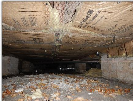
**Damaged / notched foundation support beam (North exterior beam between front porch and living space).** Although no evidence of beam sagging, cracking or movement was observed, further evaluation and repairs are recommended as necessary.
