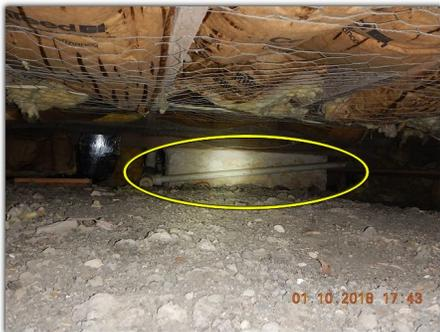
**Improper drain trap installation** (*downstairs half bathroom sink*). The drain trap for this sink was observed to be more than 24 inches from the sink and is an improper S trap, prone to siphoning. Lastly, the trap is located in the crawlspace without insulation.
