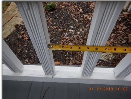
**Evidence of previous settlement / movement and deteriorated materials at front and side porch structures (multiple locations).** Further evaluation and repairs are recommended where necessary to prevent further movement or material deterioration.
