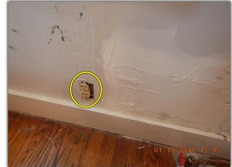
**Ungrounded receptacle(s) observed** (*one receptacle in the rear office area*). Ungrounded receptacles can be potential shock hazards or cause damage to appliances/equipment plugged into these receptacles. Grounding repairs are recommended where necessary for improved safety.
