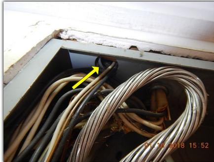
**Metal panel box not properly bonded to the electrical grounding system** (*ground bond strap observed to be detached from the grounding bar*). Further evaluation and repairs are recommended by a qualified electrician for improved grounding and safety.
