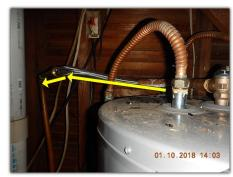
Ungrounded electric water heater (upstairs unit). Further evaluation and repairs are recommended for improved safety.
