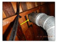
Flexible gas line connector passing through appliance case (upstairs unit). This application is not permitted as current standards require a small section of hard pipe to run through the furnace cabinet wall, prior to connecting to the flexible connector. This helps prevent vibration damage to the flexible gas line connector. Repairs are recommended by a qualified plumber for improved safety.
