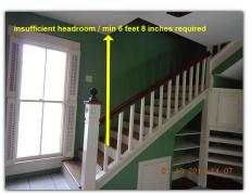
Loose / leaning newel post and handrail (smaller stairway near North entrance). Repairs are recommended.
