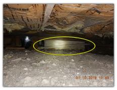
Improper drain trap installation (downstairs half bathroom sink). The drain trap for this sink was observed to be more than 24 inches from the sink and is an improper S trap, prone to siphoning. Lastly, the trap is located in the crawlspace without insulation.
