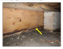
Missing hangers and poor support at opening in floor framing (where older in-floor furnace is located at North side of home). Although no evidence of movement or sagging was observed at this portion of the floor structure, monitoring is recommended.
