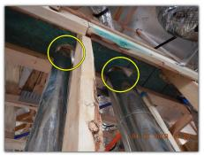
Protective metal plates are required at the wall studs where wiring bored through the studs is less than 1-1/4 inch from the face of the stud. Further evaluation and repairs are recommended where necessary to prevent possible wiring damage during drywall installation.
