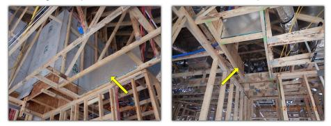
NOTE: Upon departure from the inspection, workers had arrived to deliver drywall to the property. This entailed them cutting the exterior sheathing at the rear. Ensure that the sheathing is properly sealed / repaired prior to masonry installation.
