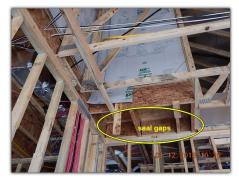
• Multiple holes and gaps were observed in the wall top plates and at portions of solid fireblocking that have yet to be sealed with an approved fire sealant foam, to include:
