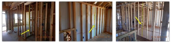
Additional blocking / support is recommended for a section of the loose / sagging sub floor at the upstairs landing.
