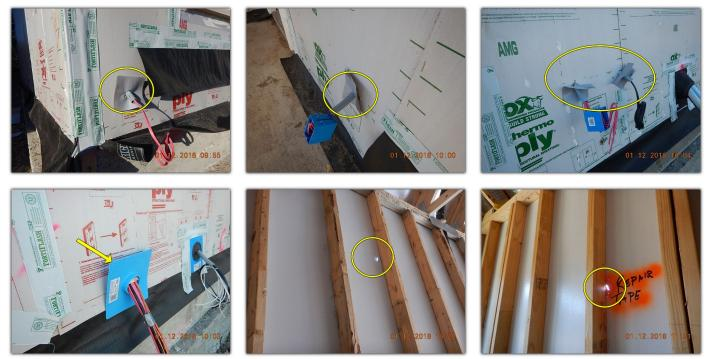
Some of the foundation anchor straps were observed to be close to the edge of the foundation, exposed and not fully embedded in the concrete, as required by the manufacturer. Furthermore, some of the straps and interior hold-down anchor straps were observed to be missing fasteners (*Check all as some straps were taped over and could not be checked*). Further review by the strap manufacturer or a qualified engineer is recommended prior to proceeding with exterior masonry.
