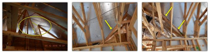
Numerous joist and beam hangers were observed to be missing fasteners. All nail holes at these hangers are to be filled with the required fasteners. Further evaluation and repairs are recommended where necessary (check all).
