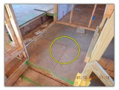
Improper sub floor nailing was observed at various locations upstairs. The sub floor material is required to be nailed every 6 inches along the edges and 12 inches along the field of the sub floor sheets. Proper nailing helps to resist subfloor "squeaking" and movement over time. All uneven sub floor edges shall also be ground or sanded down for even transitions. Further evaluation and repairs are recommended.
