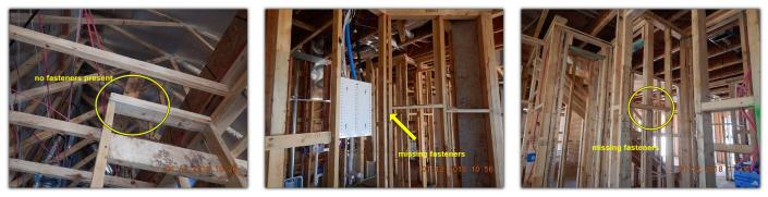
The doorway into the laundry room was observed to be improperly nailed off and is bowed. Further evaluation and repairs are recommended (proper blocking prior to nailing).
