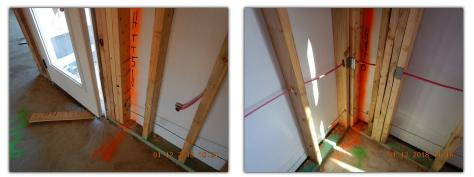
• Fastener spacing at the exterior Thermo-Ply sheathing was observed to exceed 3 inches on center at various locations. Further evaluation and repairs are recommended where necessary to ensure that the sheathing materials are properly secured to manufacturer specifications.
