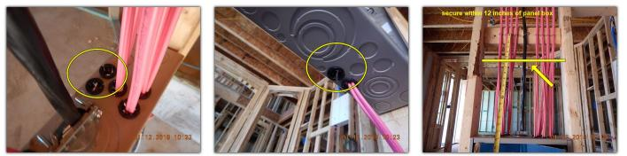
• Numerous wall intersections were observed to be missing fasteners and were not properly supported or secured (top plate at half wall coming in from garage / various wall intersections / etc.). Check all fastening requirements, according to plans, and repair where necessary.
