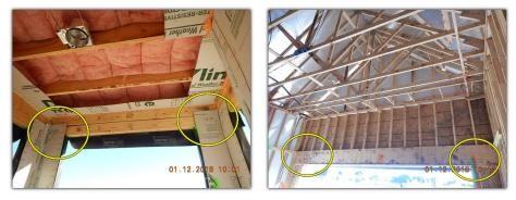
• Missing interior hold-down anchor straps were observed to be missing at various locations. Review building plans install the appropriate anchor straps, where required, prior to proceeding.
