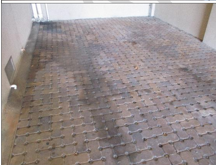
Photo #33: Some depressions were noted in the rear permeable paver parking.
