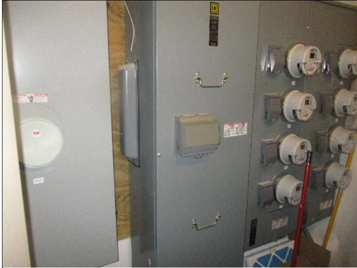
Photo #25: Electrical metering and switchgear.
