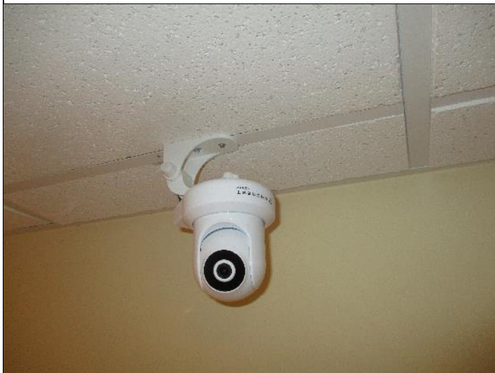
Photo #14: We noted cameras throughout the building. No camera monitoring station was discovered during our walkthrough.
