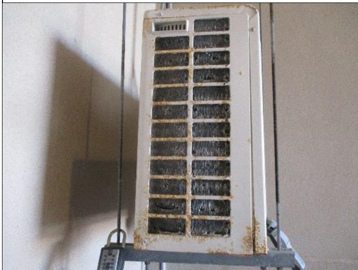
Photo #29: Deterioration noted in the mini split outdoor unit casing. Preparation should be made to replace the unit in the near future.
