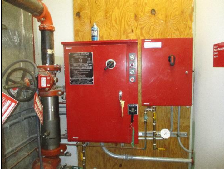
Photo #22: Fire pump controller.
