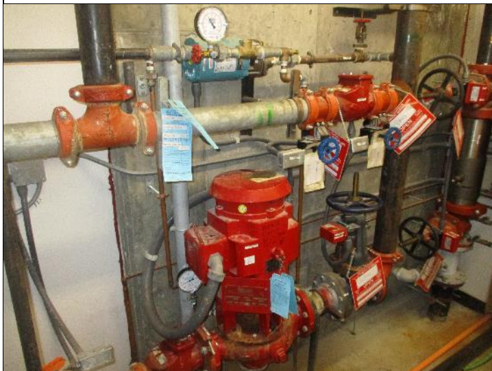
Photo #23: Fire pump with jockey pump.
