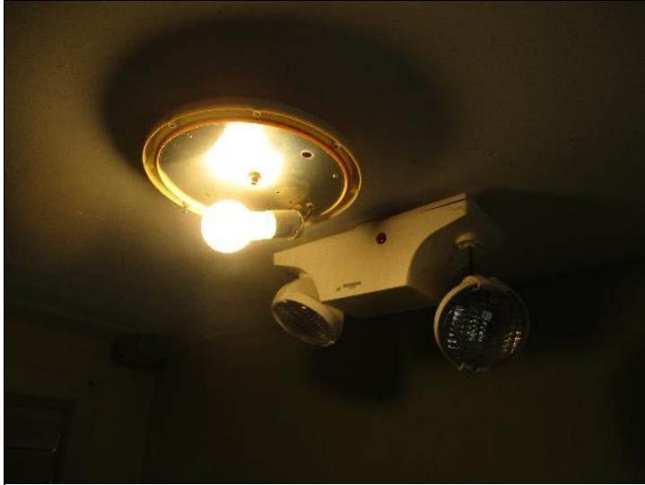
Photo #7: Missing lens noted at the bottom floor of the rear egress stairwell.
