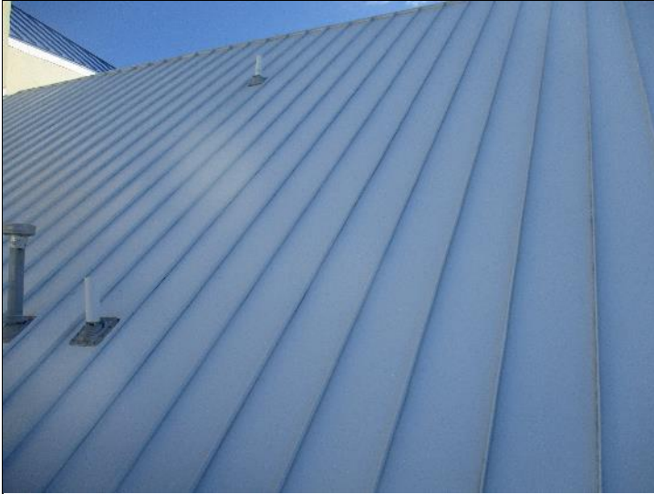
Photo #10: Standing seam metal roof.
