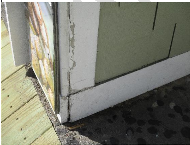
Photo #36: Minor deterioration noted in the wood trim at the boardwalk egress.
