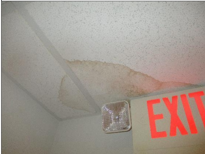
Photo #20: An apparent leak was noted in the storage area ceiling. We recommend this be monitored and repaired as needed.
