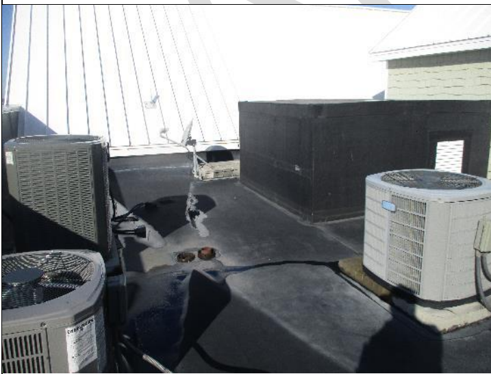
Photo #12: Building EPDM roofing.
