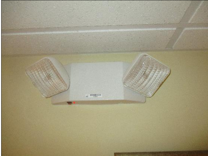
Photo #4: There were inoperable emergency lights noted during our review. We recommend they be tested and replaced where needed.
