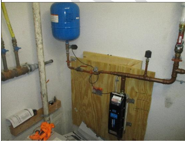
Photo #21: Domestic water inline pressure pump and expansion tank.
