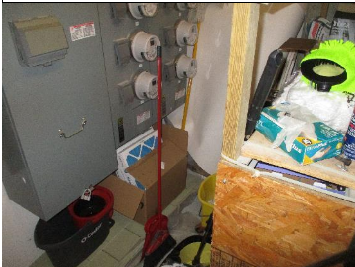
Photo #26: Electrical code prohibits storage of items within 36" of electrical equipment.
