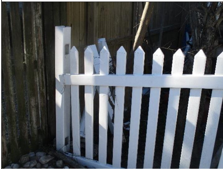
Photo #38: Damaged vinyl fencing.
