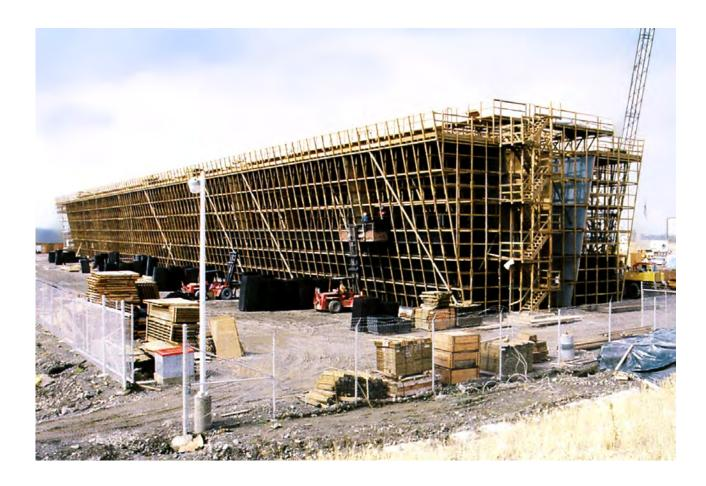
The diagonals brace the structure and carry loads to heavy-duty, hot dip galvanized anchor castings. The anchor castings transmit wind and/or earthquake loads from the structure directly into the foundation.
