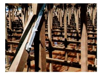
Transverse fan deck and hot water basin girts are  $2" \times 6"$ —all other transverse girts and all longitudinal girts are  $2" \times 4"$  except where loading may require  $3" \times 4"$ . Transverse and longitudinal girts are spaced on 6'-0" vertical centers. Girt lines are through bolted to the columns.
