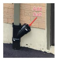
This system was tried and tested with good results in the previous two winters, with salt applications not required. Nevertheless, be on the lookout for pipes freezing over. If you find ice formation in the Wye-joint, you can first pour boiling water into the opening before then adding the salt to do its work to melt the ice.
