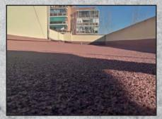
Waterproof and spray-applied membrane made of recycled rubber
