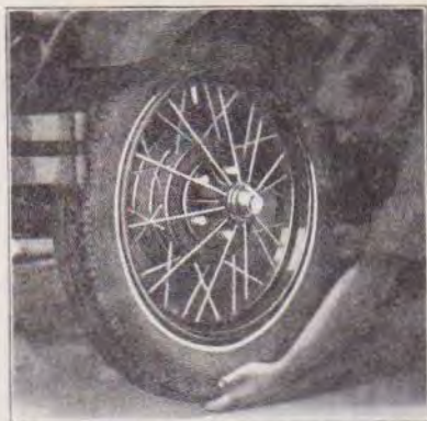
Figure 26 Centering Tire on Rim
