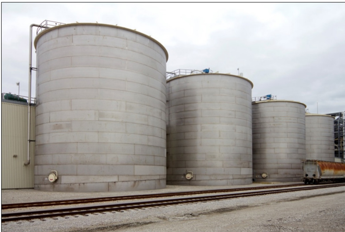
Figure II.12. Ethanol Fermentation Tanks.
