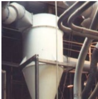
Cyclone Dust Collector (Source: OTI)
