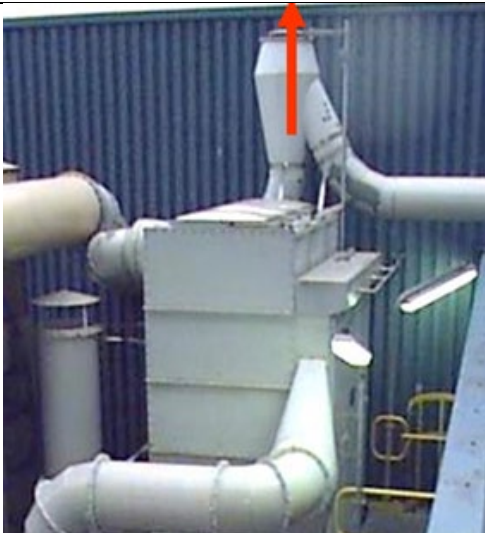
Flame Front Diverter (Source: J.O.A.)
