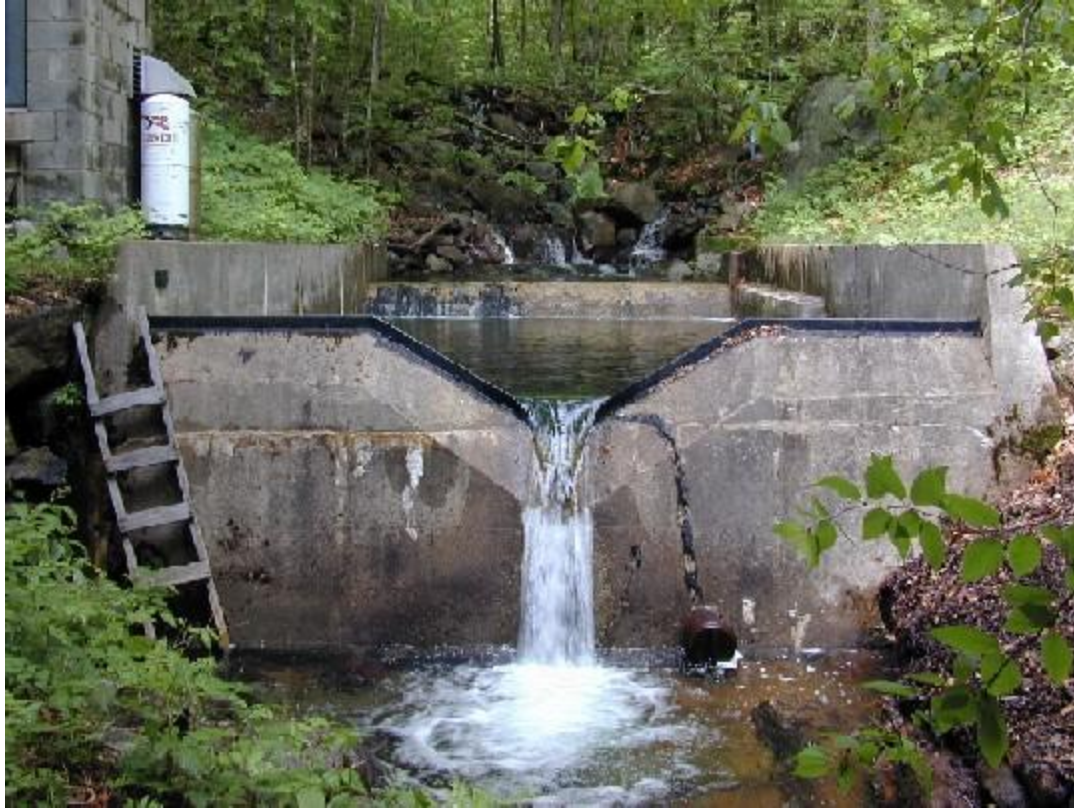
Figure 42. V-notch weir.
