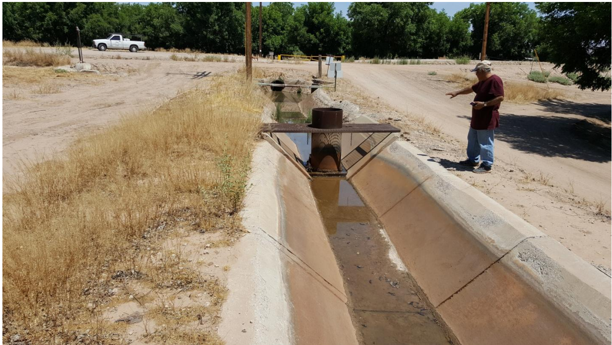
Figure 18. Trapezoidal flume in southern New Mexico Irrigation canal located at GPS coordinates: 32.391389, 106.846111.
