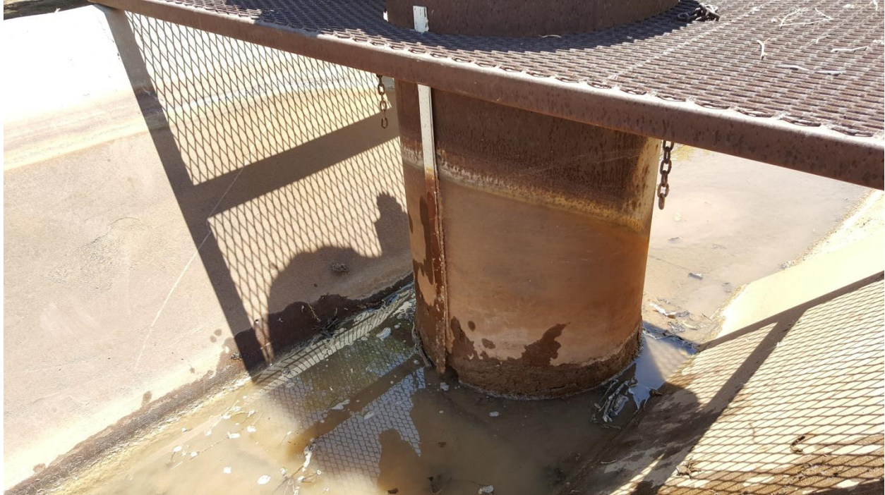
Figure 19. Close up (upstream side) of previous flume, with visible rust patterns indicating maximum water height and critical flow profile.
