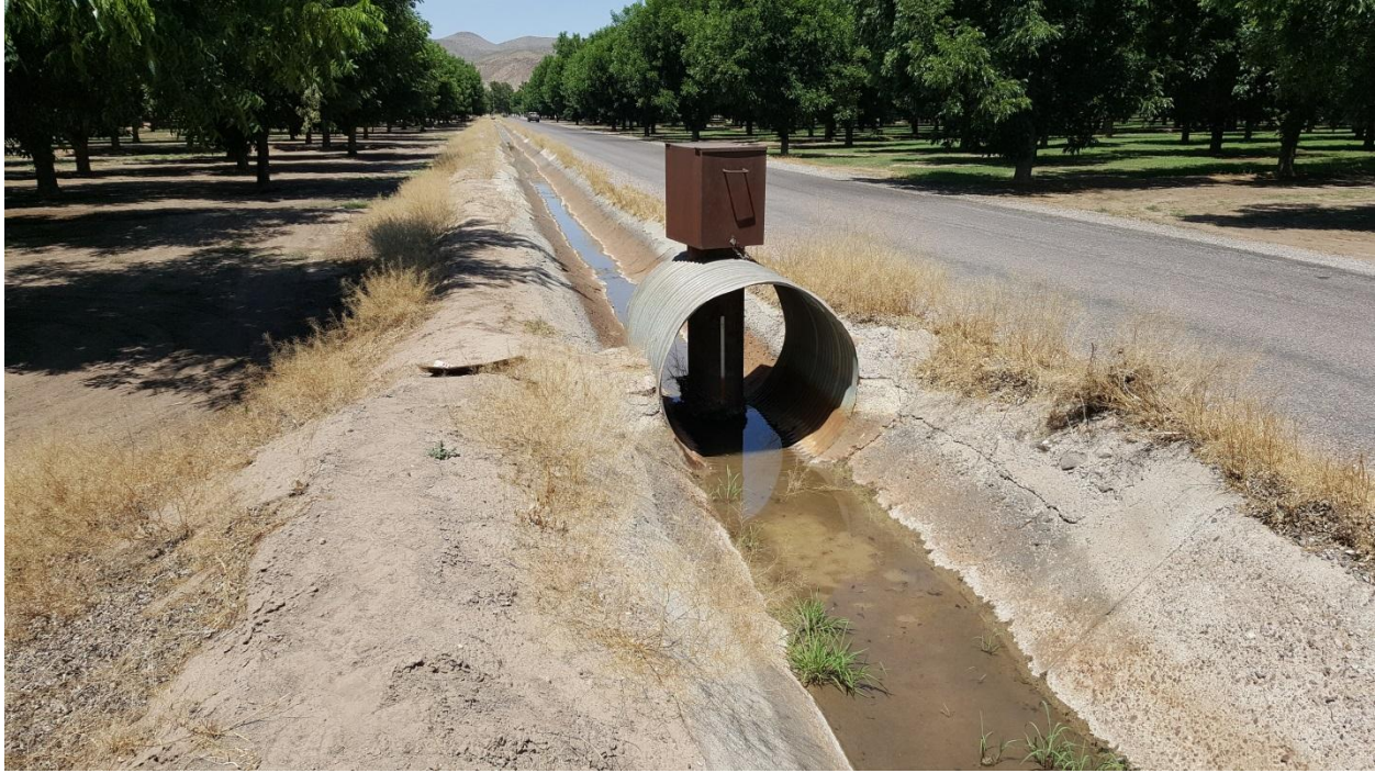
Figure 3. Circular flume in southern New Mexico irrigation canal, located at GPS coordinates: 32.359167, 106.784722.
