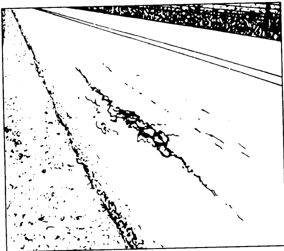
Figure 16-10.—Edge cracks.
