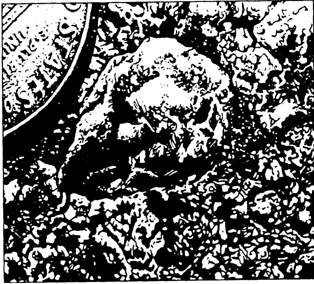
Figure 16-24.—Polished aggregate in pavement surface.
