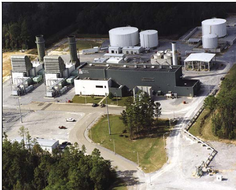
Figure 18. 110 MW CAES Plant in McIntosh, AL
