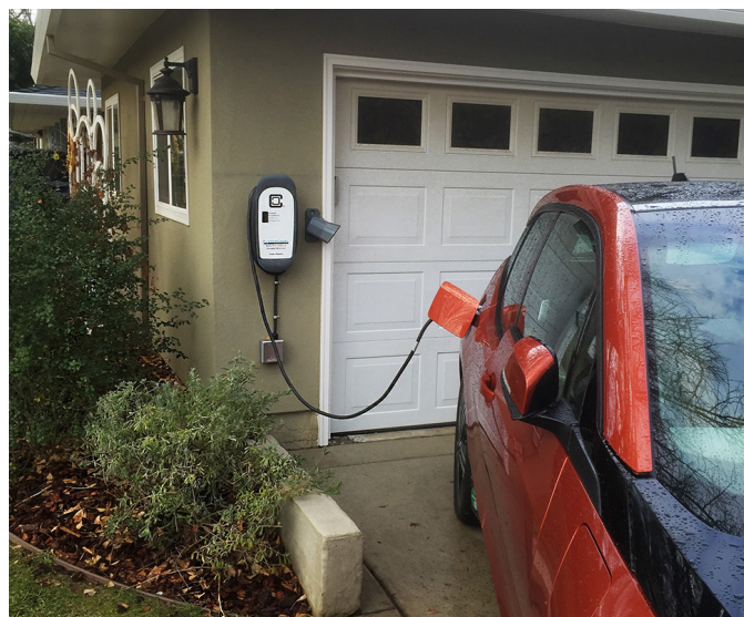
EVSE installation. Source: Clipper Creek
