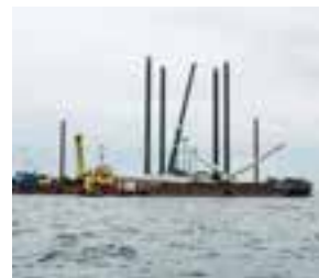
Clearing the site
