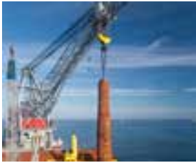
Site preparation and civil works
