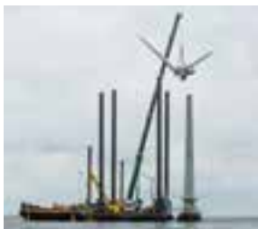
Dismantling the project
