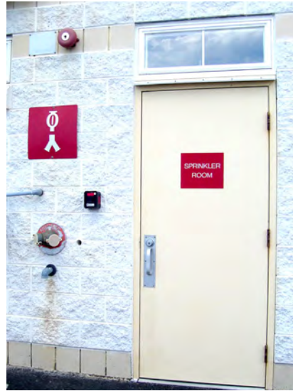
Figure 8.7. The sign on this door indicates that a sprinkler control valve is located within the room.
