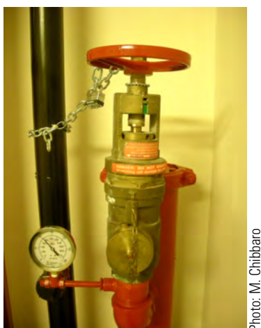
Figure 9.6. An FHC equipped with a pressure-regulating device.
