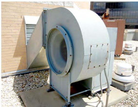
Figure 12.12. A stair pressurization fan.
