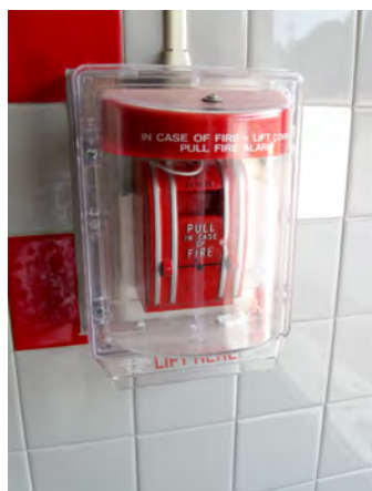
Figure 11.8. A manual pull station cover.
