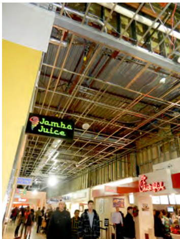
Figure 13.9. An occupied area of an existing shopping mall being renovated. Apparent deficiencies include a suspended ceiling grid without ceiling tiles, detectors and sprinklers at the future ceiling level, and protective caps on sprinkler heads.
