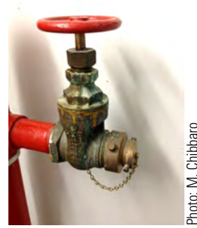
Figure 9.7. A 2½" threaded FHC. The valve is opened and closed with the red hand wheel. The hose outlet has a 2½" by 1½" reducer to facilitate the use of different hose sizes. The 1½" cap is attached to the valve body by a chain.
