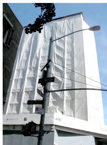
Figure 13.16. A temporary barrier covering an entire building.
