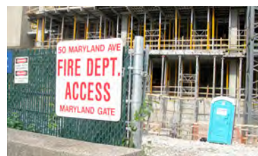
Figure 13.5. Temporary fire apparatus access.
