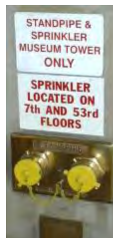
Figure 10.16. An FDC sign showing partial system coverage.
