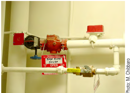
Figure 8.2. A sprinkler zone control station. The sign on the control valve indicates “first floor south” but there is no indication where the boundary is between south and north.
