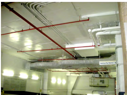
Figure 8.1. A fire sprinkler system.
