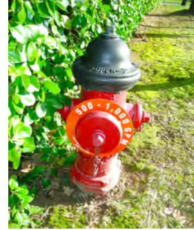
Figure 4.8. A fire hydrant with flow indicator sign.
