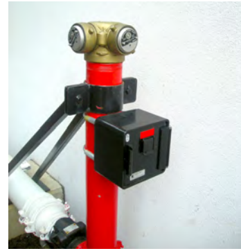
Figure 10.6. An FDC with locked plugs. The key is in the key box below the inlets.
