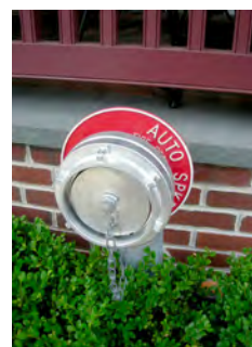
Figure 10.5. A quick-connect type of FDC.
