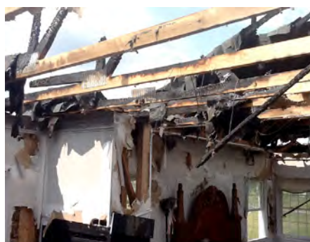
Figure 7.8. Wood trusses after an attic fire.
