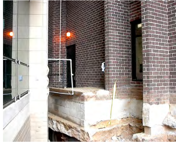
Figure 13.10. An exit discharge area from an occupied building. The path to safety was demolished during adjacent construction.
