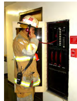
Figure 11.13. A fire officer speaking into the main handset at the control panel for a fire department communication system. This panel also houses the portable handsets used by firefighters at remote jacks.
