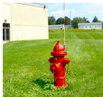
Figure 4.7. A dry barrel fire hydrant.
