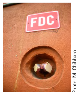
Figure 10.13. An FDC recessed into a wall. Note the notch on left prevents hose lines from kinking.
