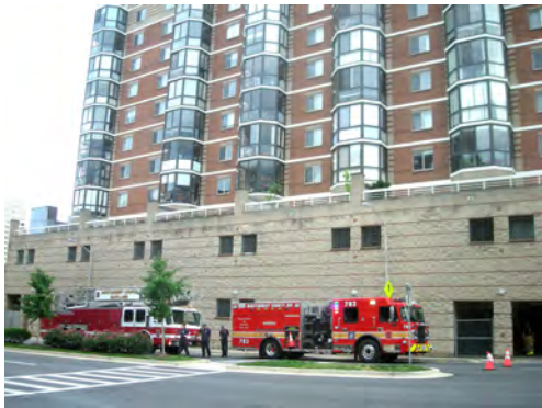
Figure 11.12. This high-rise building has three garage levels interconnected by open vehicle ramps. Those three levels have a single occupant notification zone.
