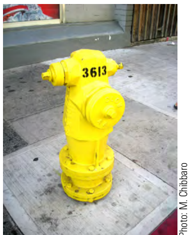
Figure 4.6. A wet barrel fire hydrant. The operating nut for the small hose outlet is on the right. The operating nut for the large outlet is on the rear of the hydrant.
