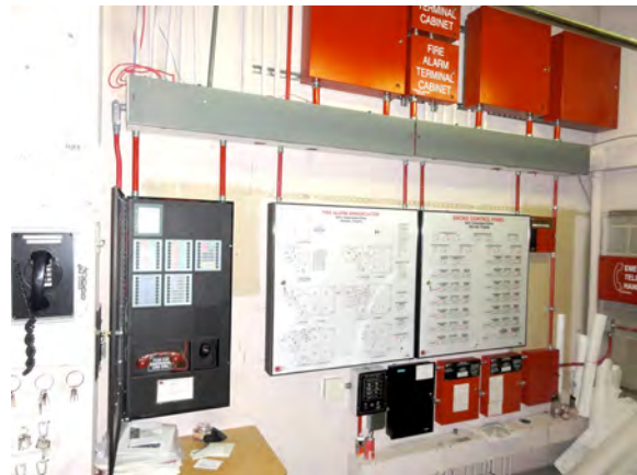
Figure 11.15. The inside of a fire command center.
