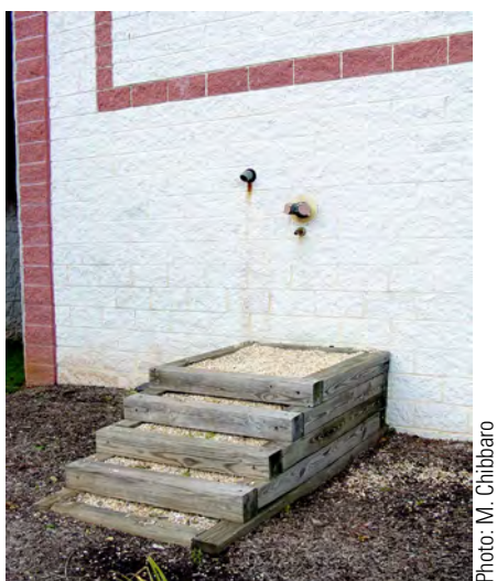
Figure 10.12. A platform built up to reach an FDC. This creates an unnecessary fall hazard.
