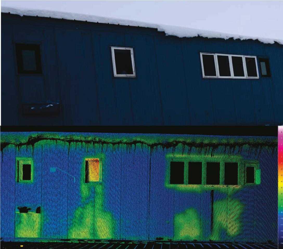
Figure 18. East face of GWR, displaying significant heat loss and insulation damage below white-trim windows. The damage to insulation continues from the top-floor windows fully down to ground level. A patched panel to the right of the windows also displays heat loss below. No significant heat loss was measured along the roofline or exterior panel seams. Temperature scale for the bottom image:  $-15^{\circ}\text{C}$  to  $5^{\circ}\text{C}$ .
