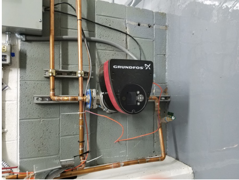
Figure 16 – DHWP-1 HPCP Model 40-80F
