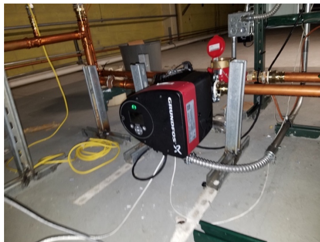
Figure 22 – AHU-19 HPCP
