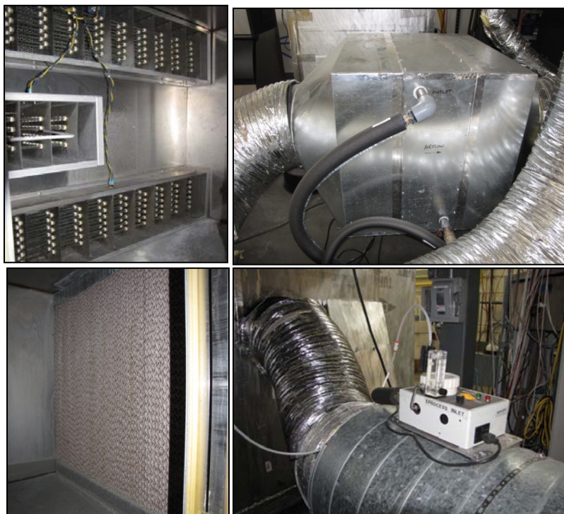
Figure 2. Duct heaters used to control humidity (top left), heat exchanger to provide cooling (top right), evaporation pads (bottom left), and temperature and humidity measurement at inlet to plenum (bottom right)
