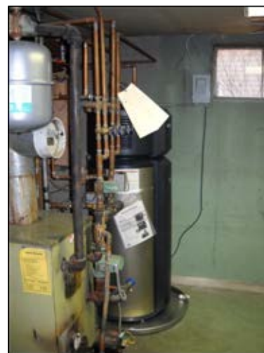
Figure 9. This HPWH benefited from the waste heat of the boiler used for space heating.
