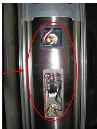
Figure 12. Both heater covers removed. The upper heater is the main heater and the lower heater is the backup (not connected).
