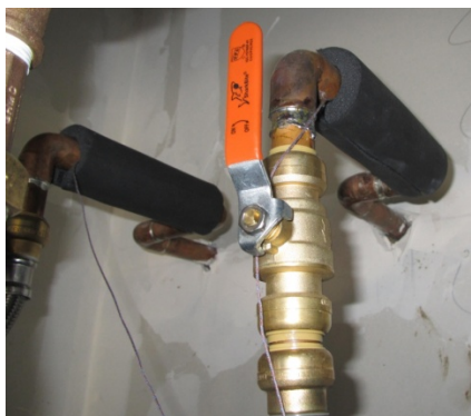
Figure 21. Pipe insulation covering the surface-mounted TCs on the inlet and outlet water pipes
