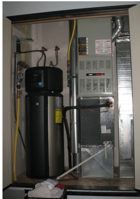
Figure 13. GE GeoSpring HPWH installed in garage closet
