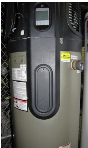
Figure 8. The A.O. Smith Voltex HPWH with the upper heater cover shown.
