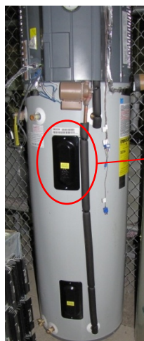
Figure 5. The Rheem HPWH with heater covers shown.
