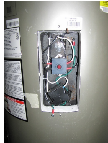
Figure 10. After the insulation is removed, the tank wall is accessible for installing a TC.
