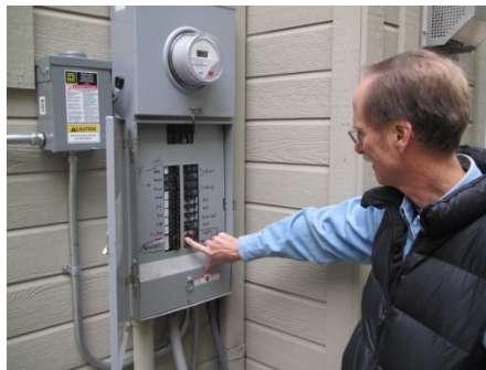
Figure 14. Turn off the breaker for the HPWH.
