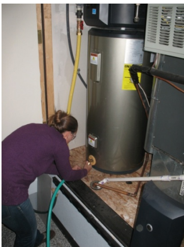
Figure 16. Connecting the hose to the drain in preparation for installing the flow meter
