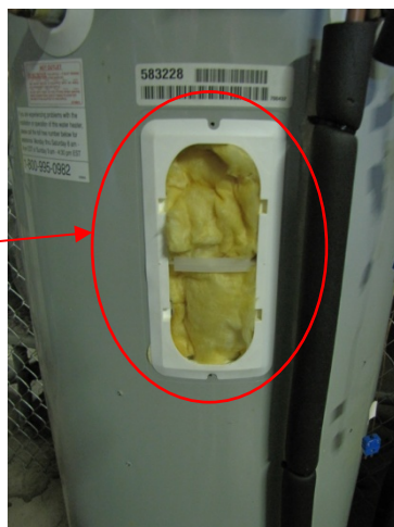
Figure 6. The top heater access point with the cover removed. The fiberglass insulation can be removed.
