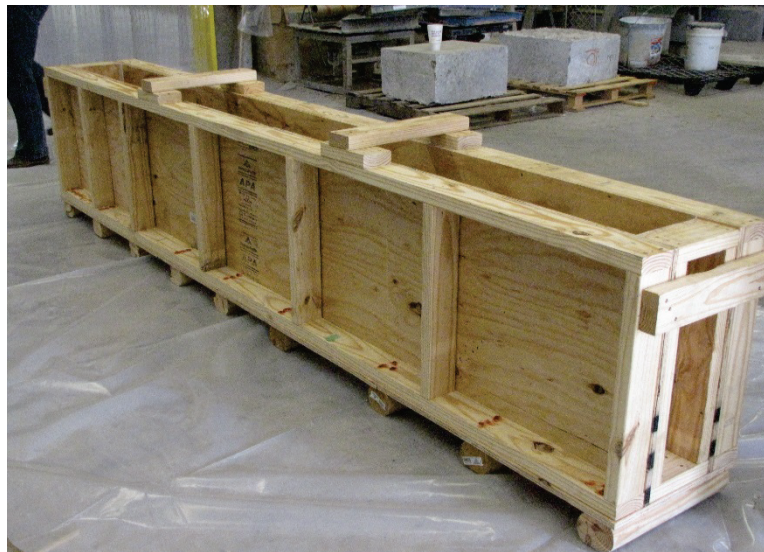
Figure 3.1. Completed formwork for beam.
