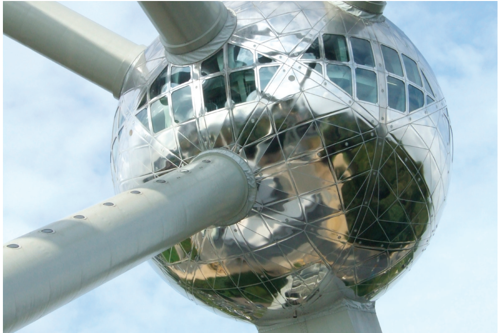
Photo 2: Atomium Brussels. The renovated spheres are now clad with sandwich panels made of 1.2 mm outer skin of X2CrNiMo17-12-2/1.4404 stainless steel grade – Brussels (B)
