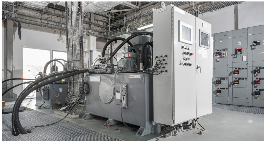
Complexity in applications or specification may require complex control packages nearly the same size as the hydraulic power unit. A well designed and built power unit not only achieves functional criteria but can also be an attractive addition to the production floor.
