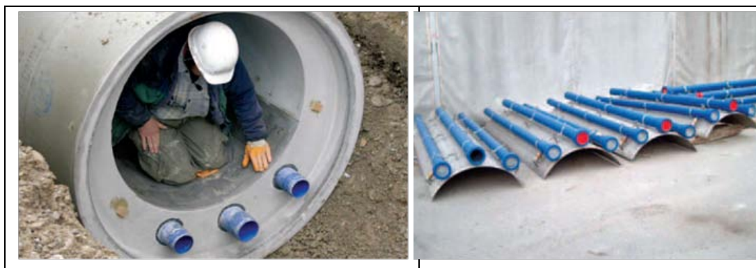
Figure B2. Integrated heat exchanger segment; (reference 2).
