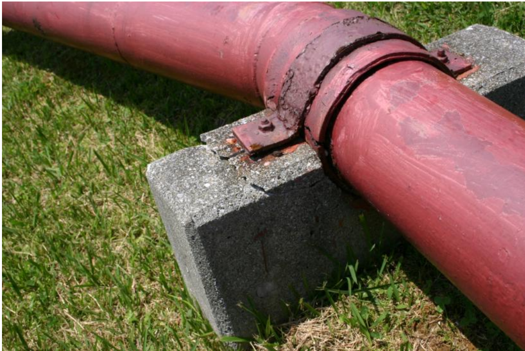
Figure B5. Photograph of the structural damage caused by corrosion of the pipe at the Chimyu-Wan Tank Farm #3, Okinawa, Japan.
