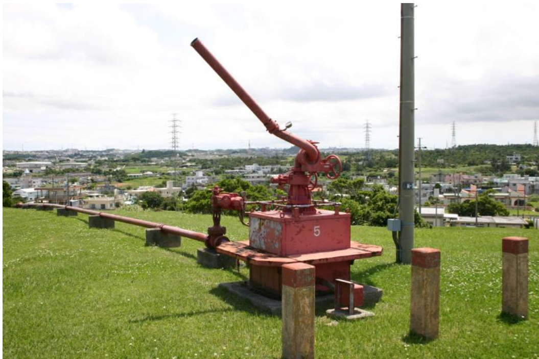
Figure B2. Photograph of the deluge system showing a water cannon and the supply pipe.
