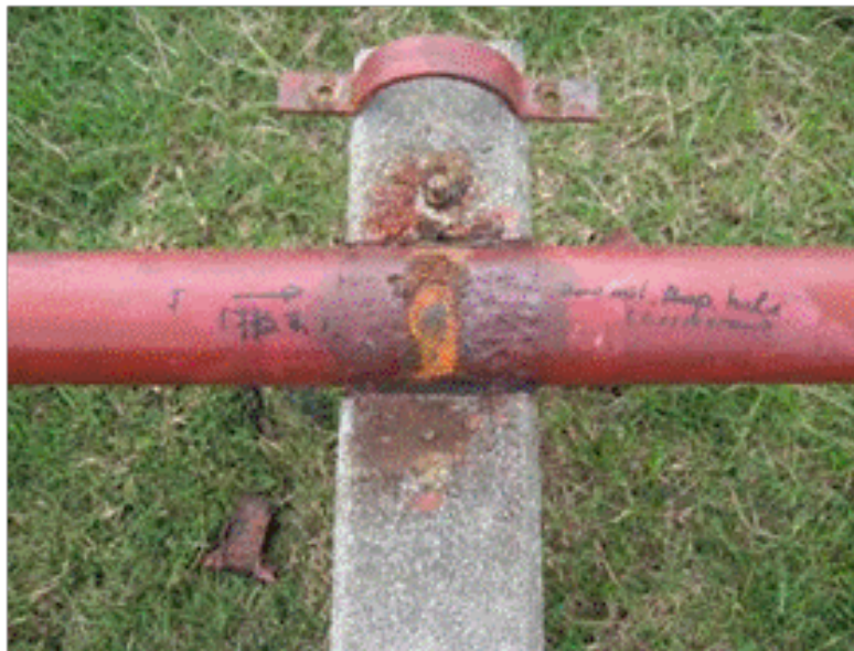
Figure 1. Severe corrosion at pipe support.
