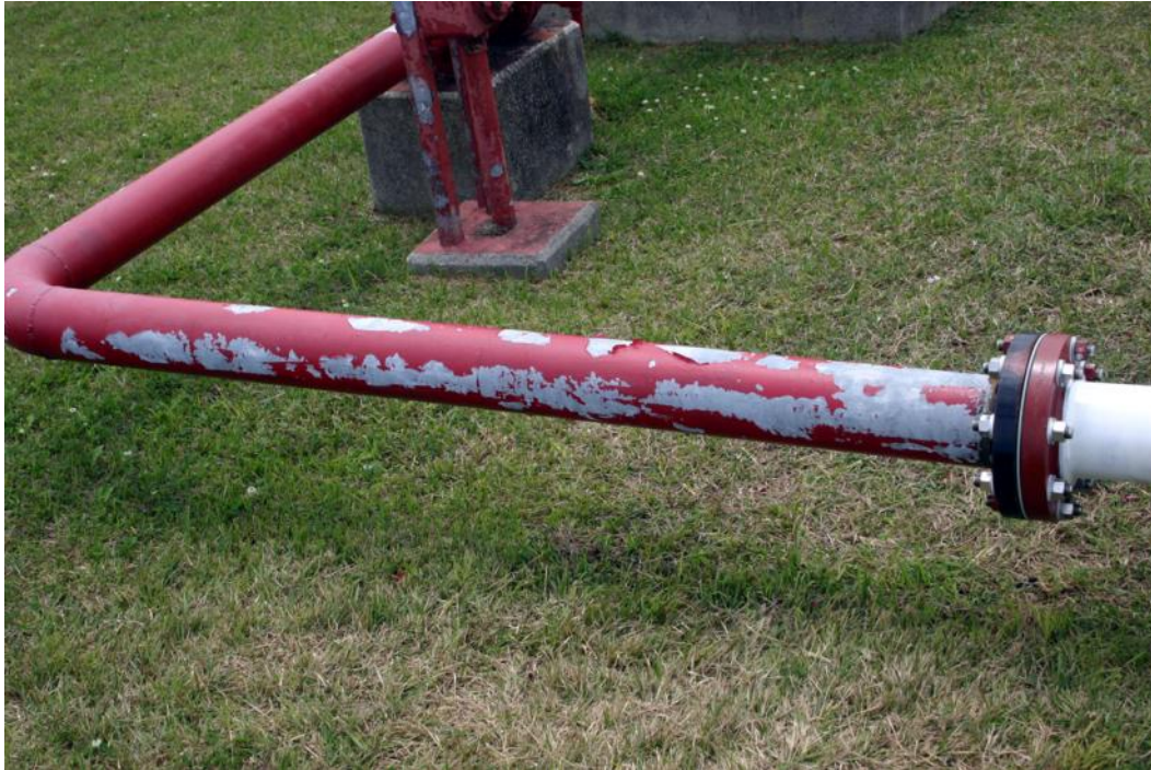
Figure B3. Photograph of the fire suppression supply pipe that was galvanized.
