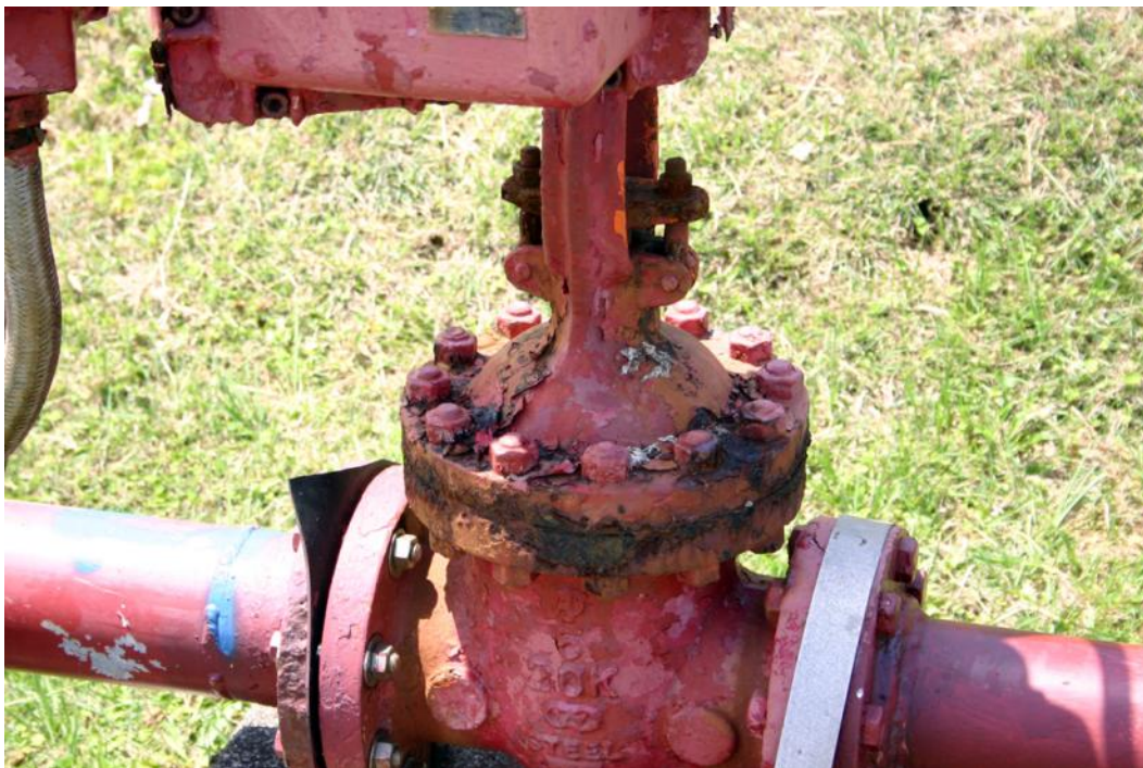
Figure B4. Photograph of one of the corrosion damaged valves that was replaced at the Chimyu-Wan Tanks Farm #3, Okinawa, Japan.
