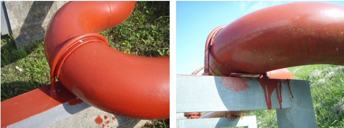
Figure 6. Two sections of installed pipe showing evidence of touch up painting.
