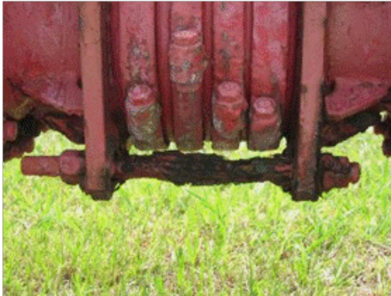
Figure 2. Severely corroded flange bolt
