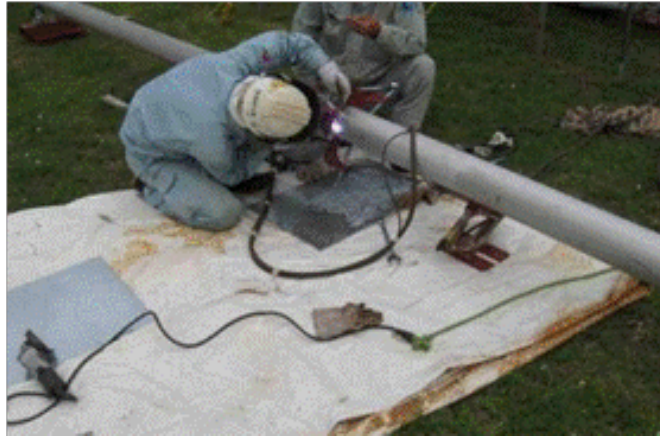
Figure 4. Arc welding replacement pipes.
