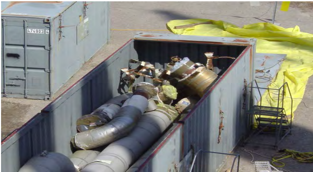
Figure 4-2. Piping with internal contamination and openings sealed with plastic and tape.
