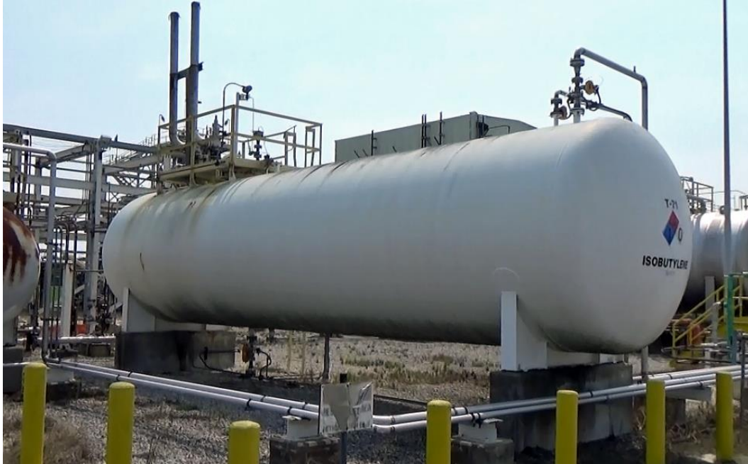
Figure 43. Isobutylene Storage Tank at the Arkema Crosby Facility. The isobutylene tank posed a concern because the controlled burn of the six refrigerated trailers in the laydown area would occur within about 40 yards of this storage tank. (Source: CSB Photo)
