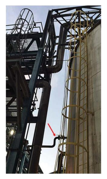
**Figure 22.** Pre-Incident Photograph of the Foul Condensate Tank. The line from the weir inside the tank to the turpentine recovery system is indicated by the red arrow. The valve at the foul condensate tank is kept open, but the valve at the turpentine recovery system (**Figure 21**) is kept closed. Photograph: PCA.
