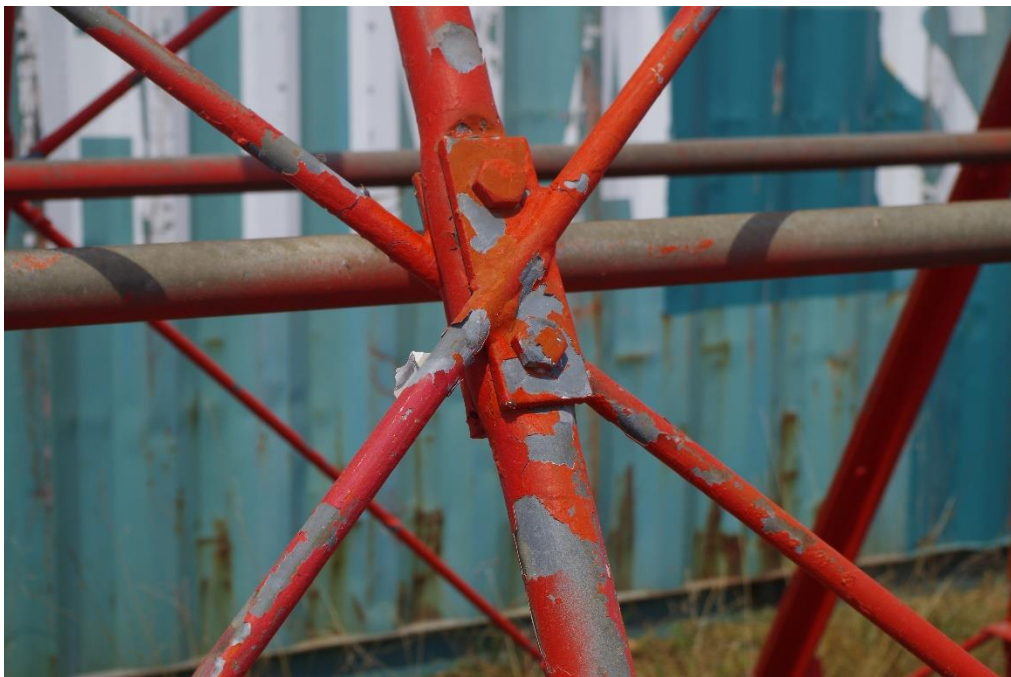
Figure 13. Bolted Connection between Diagonals and Redundant Horizontal
