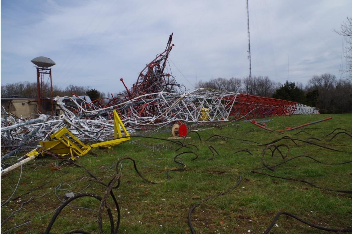
Figure 6 Top Section of Collapsed Communication Tower
