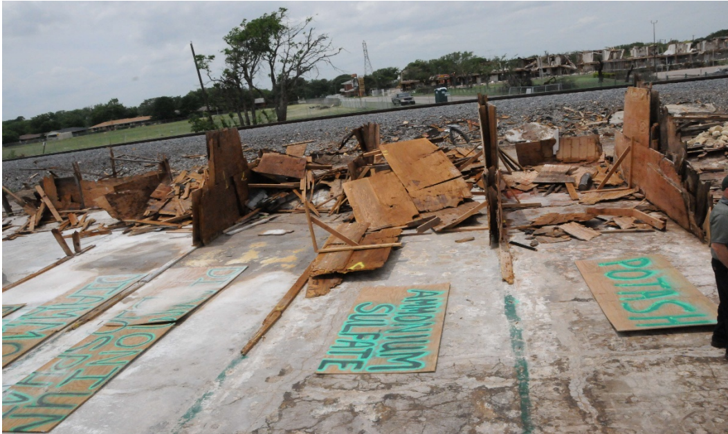
Figure 8. Plywood Bin Wall, Post-Explosion (Source: CSB)
