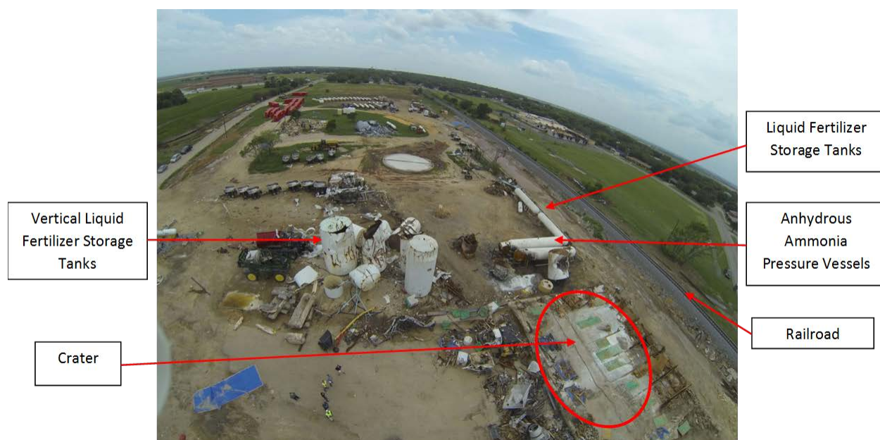
Figure 17. Anhydrous Ammonia Pressure Vessels (Source: CSB)
