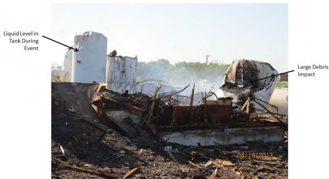
Figure 16. Liquid Fertilizer Tank Damage (Source: CSB)
