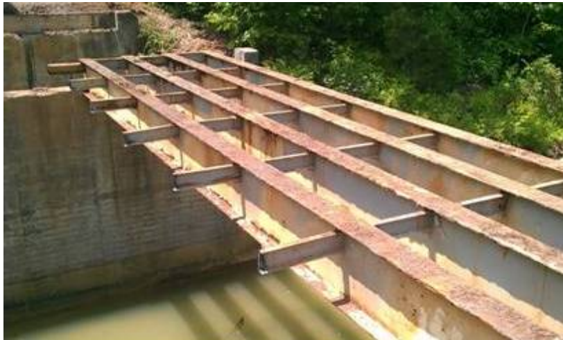
Figure 6. Corroded support beam structure visible during demolition.
