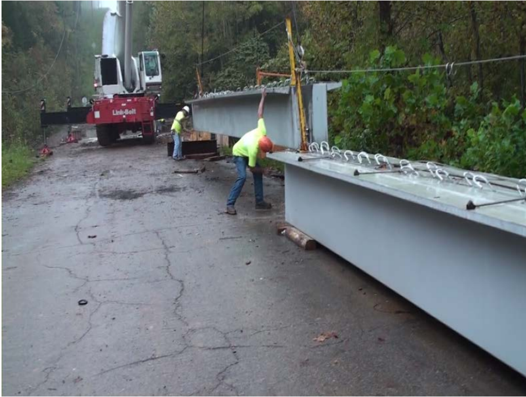
Figure 12. Crane lifting an HCB for installation.
