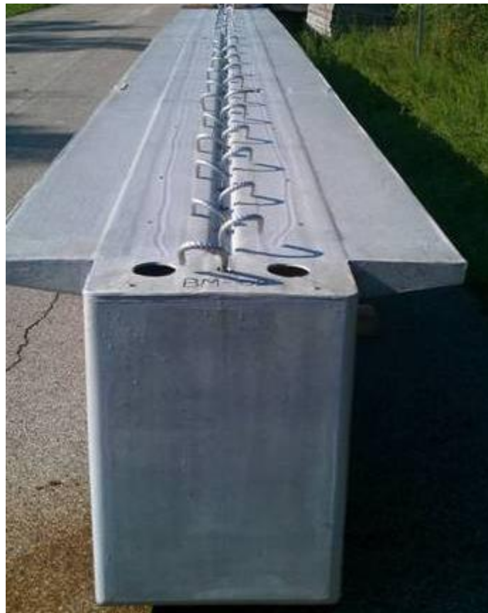
Figure 3. Ports for injecting SCC.
