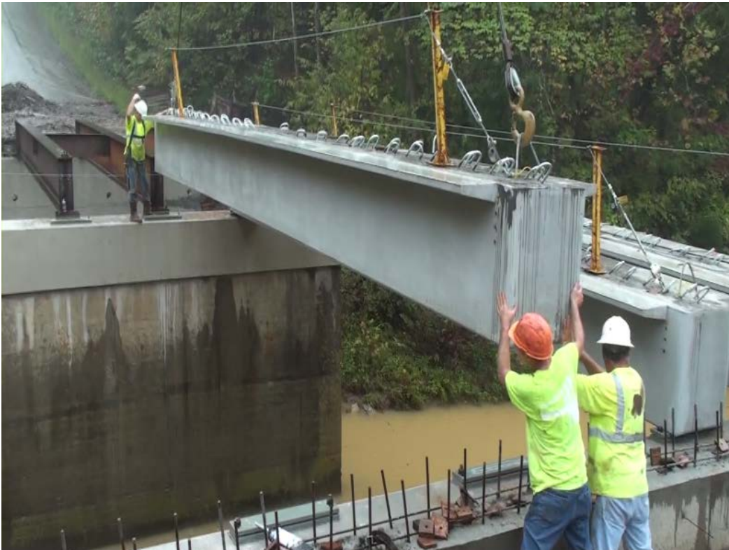
Figure 13. Placing an HCB.
