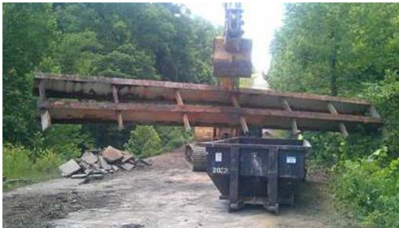
Figure 7. Lifting degraded steel beam structure during demolition.
