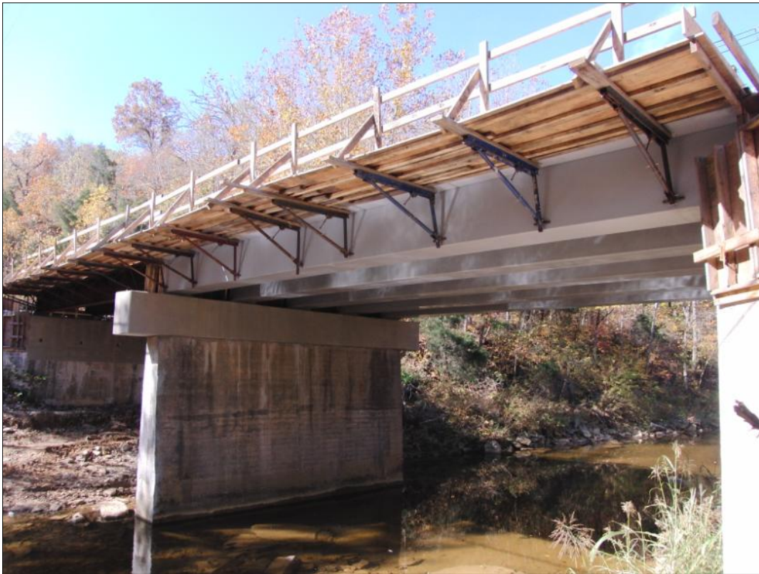
Figure 15. Bridge deck construction in progress.
