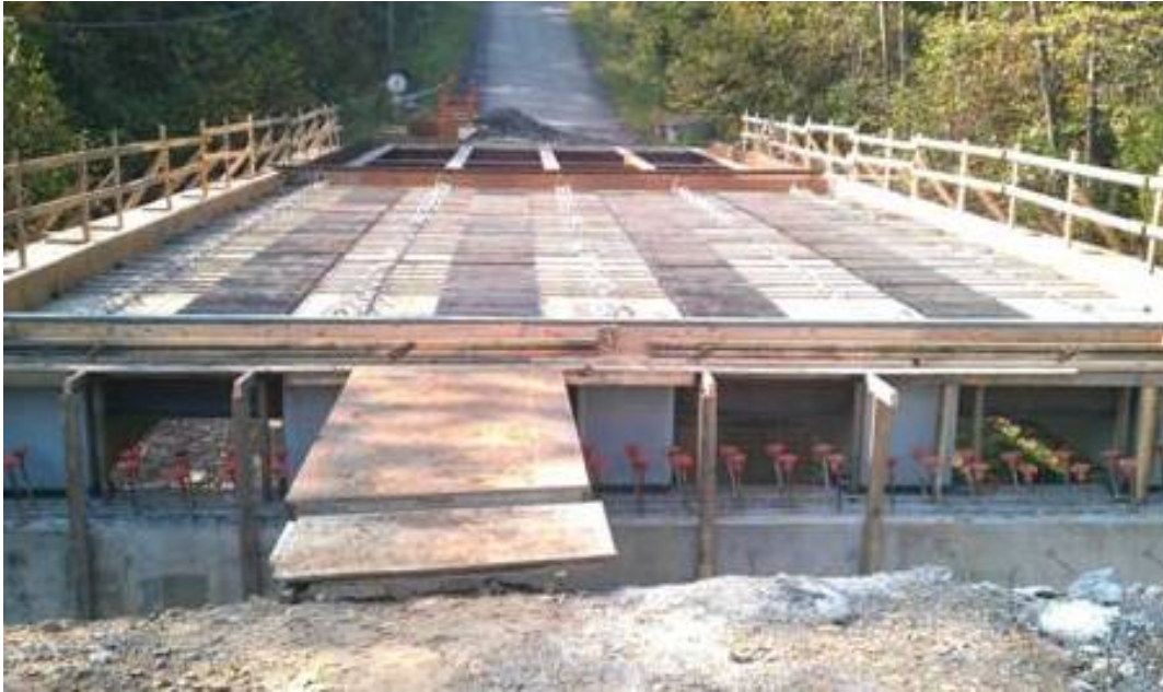
Figure 14. Forming bridge deck and installing rebar.
