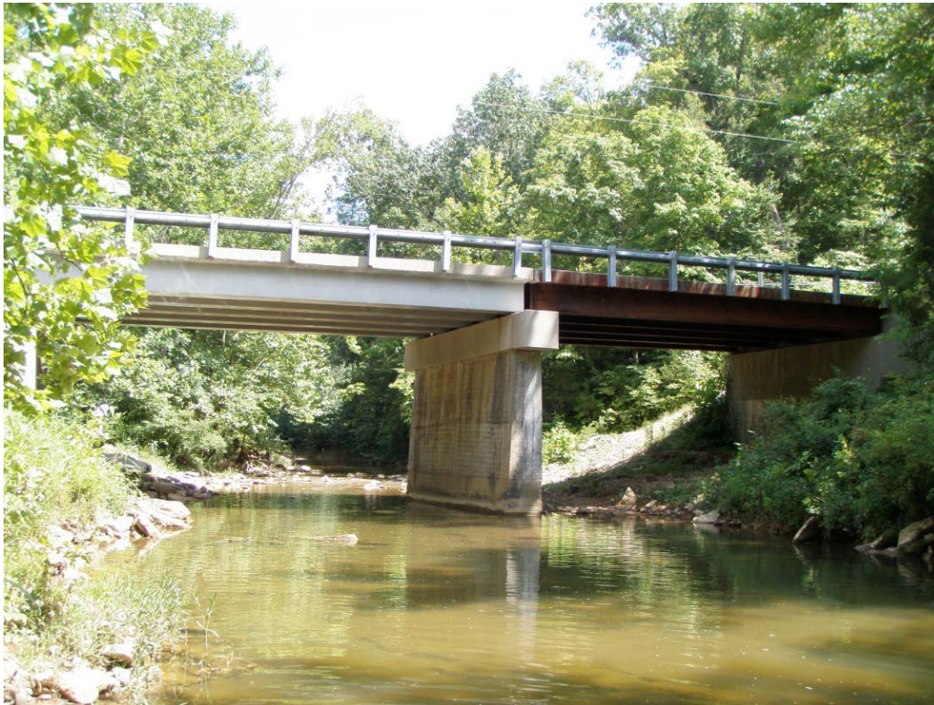
Figure 16. Completed bridge No. 4 with HCBs (left) and Gridform deck on Cor Ten® weathering steel beams (right). 1
