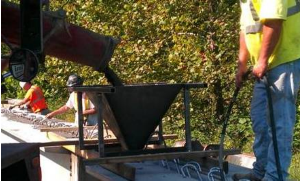
Figure 10. Casting the internal compression reinforcement arch.
