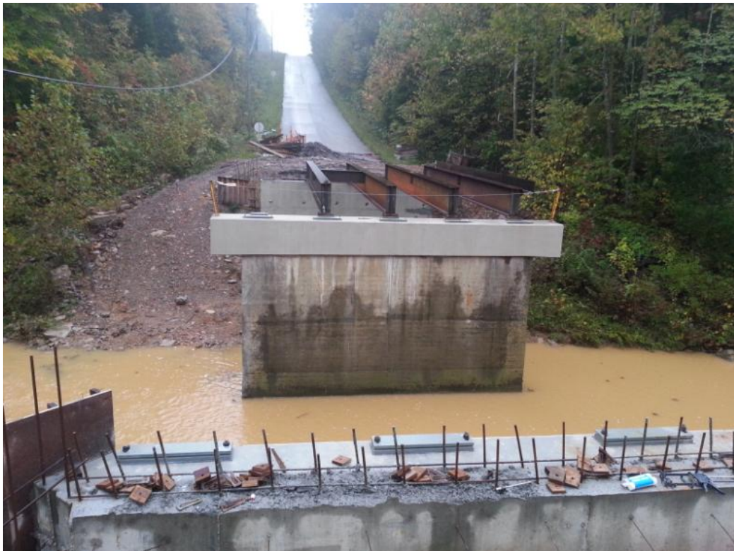
Figure 11. Span of Bridge No. 4 (foreground) prior to installing HCBs.
