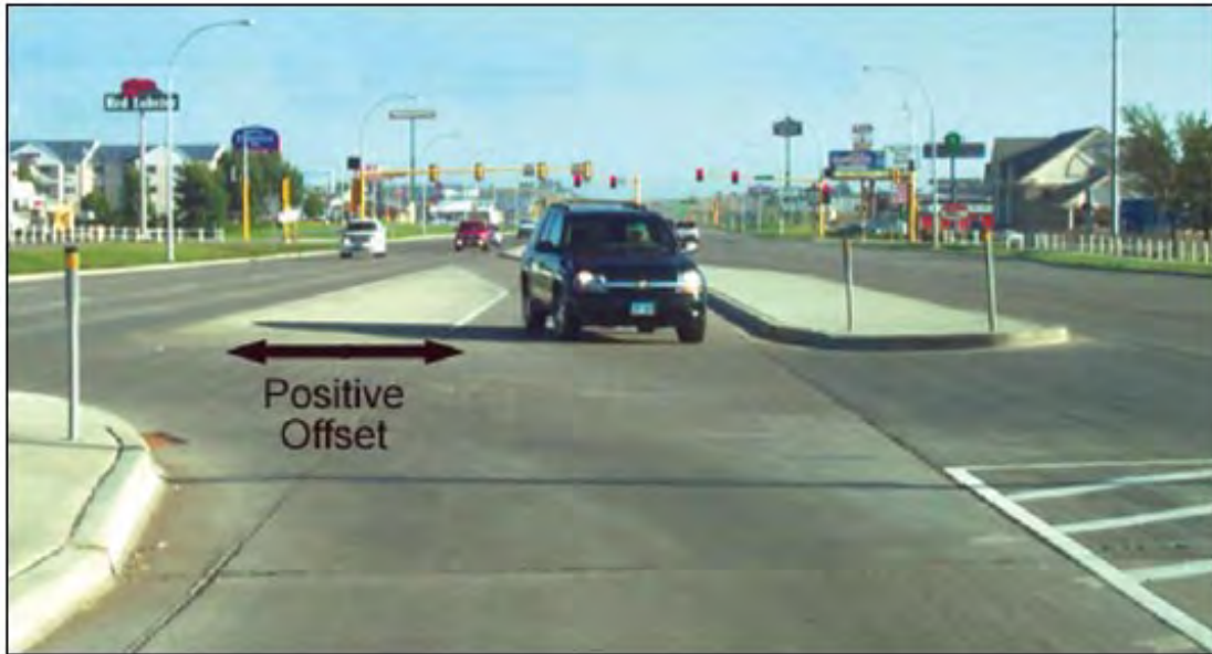
Exhibit 11-5. Example of positive offset left-turn lane.
