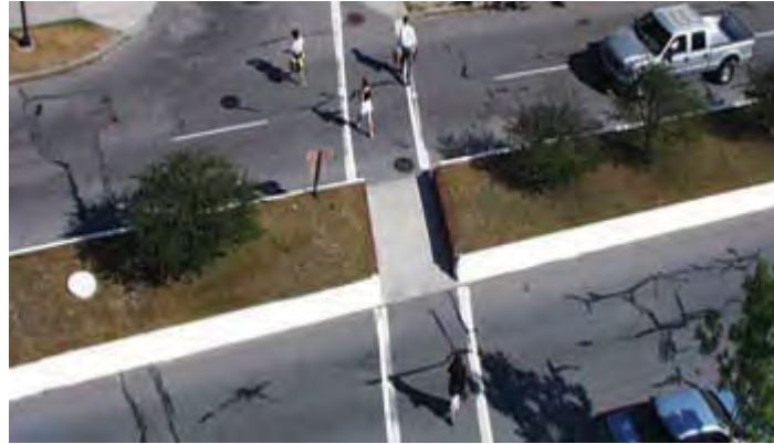
Exhibit 8-5. This refuge island enables two-stage pedestrian crossings.
