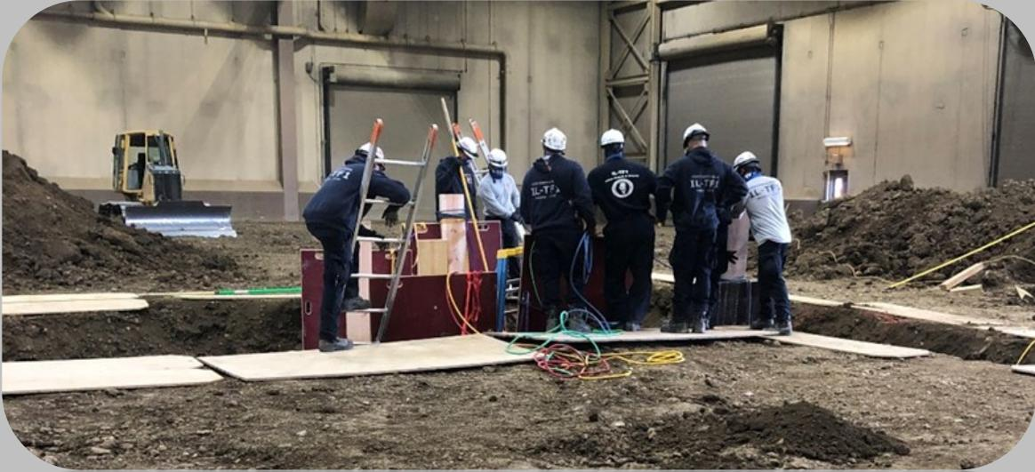
October 14 - 15 Trench Training at Operating Engineers Local 150 in Wilmington IL – TF 1 members working in “T” Trench environment, using Paratech Struts and support equipment.
