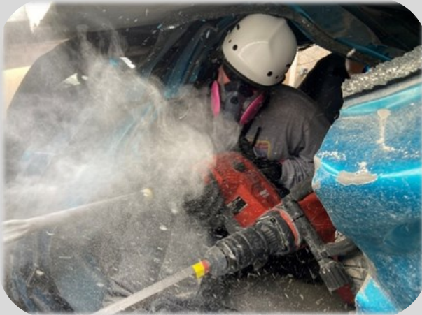
Tunneling thru a vehicle and breaching concrete
