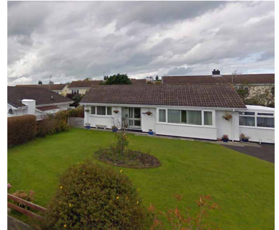
Single storey bungalows in a cul-de-sac formation at Swn-Y-Llethi
