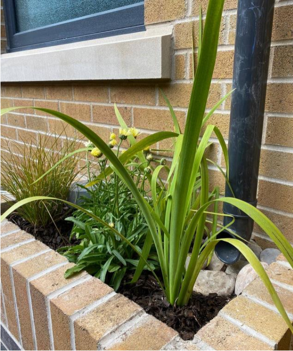
Figure 8. Example of Bio-retention planter
