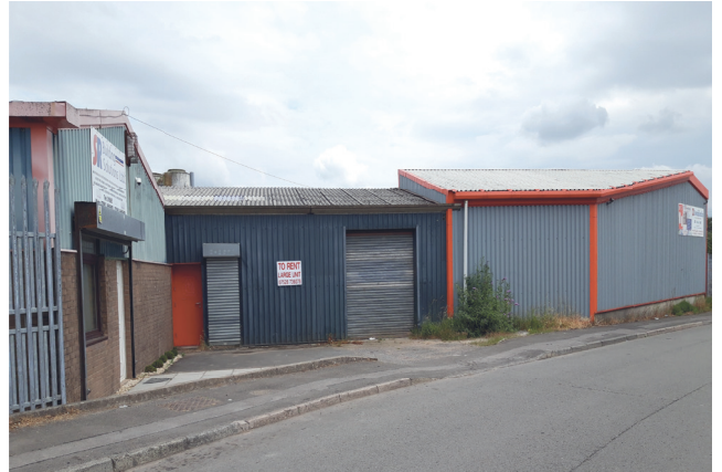
Existing units along eastern approach
