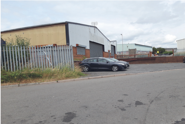
Existing units along eastern approach road
