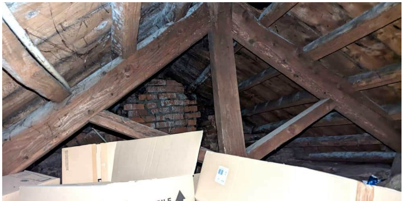
Figure 13: Softwood King-Post roof truss to the principal farmhouse range. Note the sarking-boarded roof and the rustic pole purlins.
