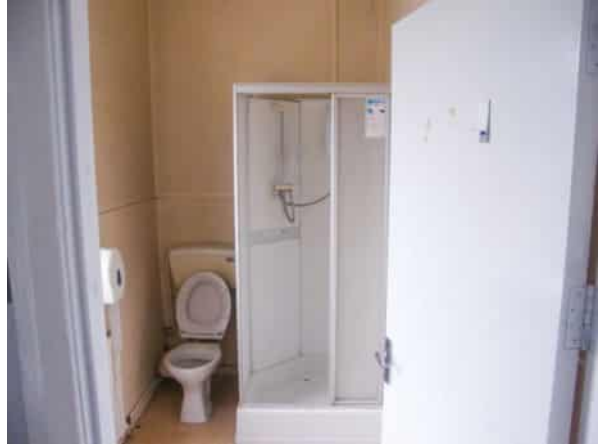
Photo 44: F3 bathroom, facing west
