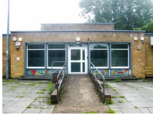
Photo 50: Principal (west) elevation of the former Magistrates' Court
