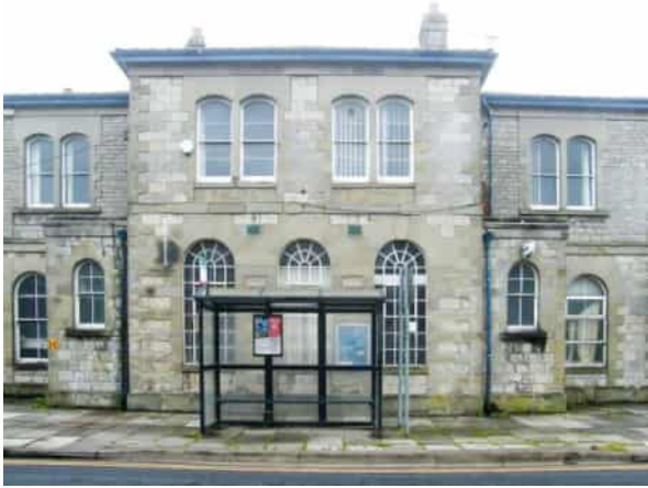
Photo 1: North elevation of Cowbridge Police Station
