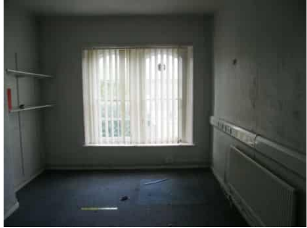
Photo 38: F1 west office, facing north
