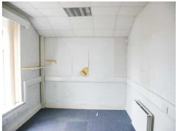
Photo 42: F2 south room, facing south
