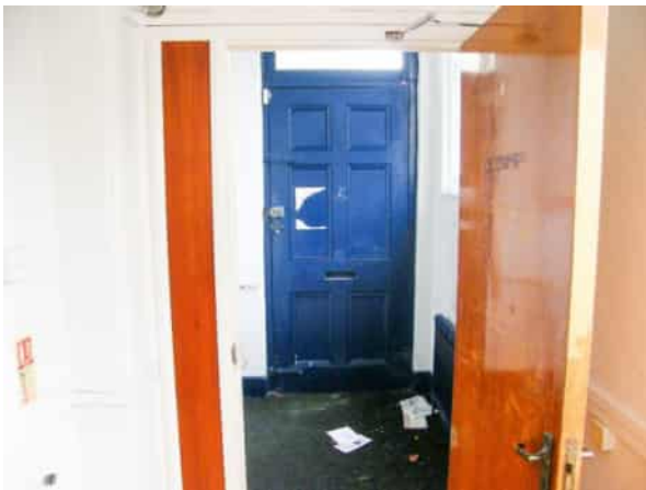
Photo 15: View from G1 into the west porch
