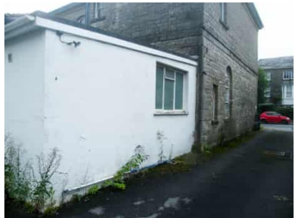
Photo 4: East elevation of Cowbridge Police Station
