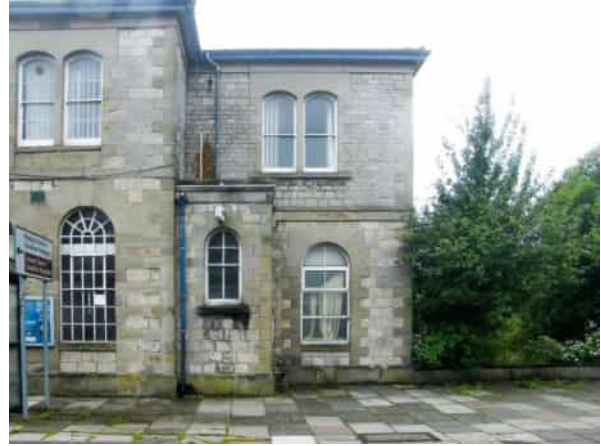
Photo 8: East wing, north elevation
