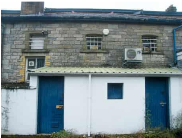
Photo 9: South elevation of the cell block
