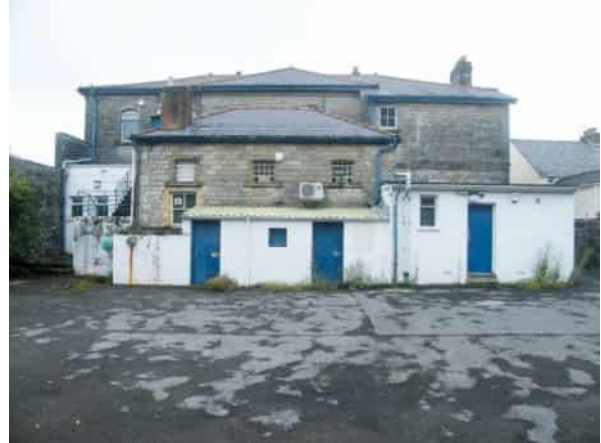
Photo 2: South elevation of Cowbridge Police Station
