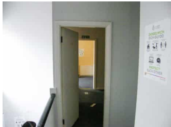
Photo 36: View west along landing
