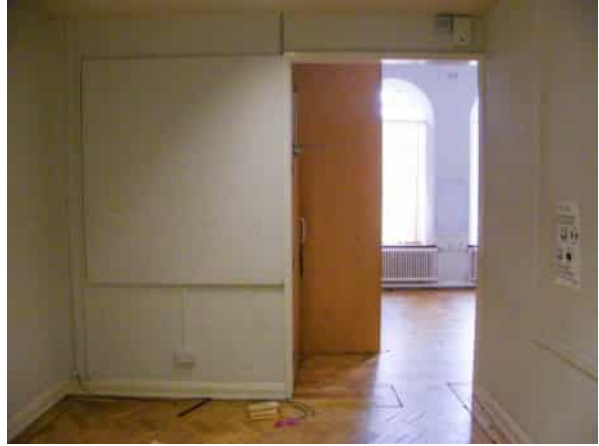
Photo 14: West side of G1, facing north
