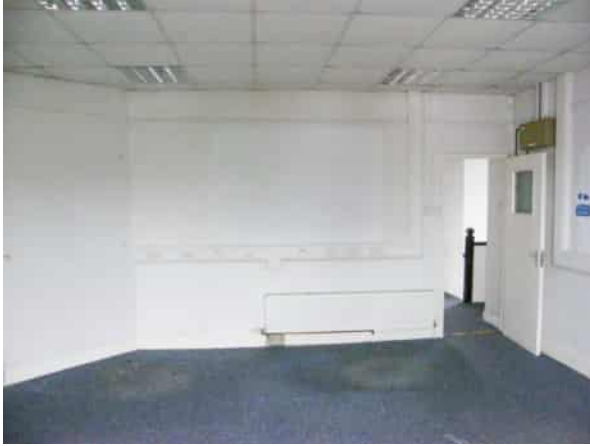
Photo 43: F2 north room, facing south
