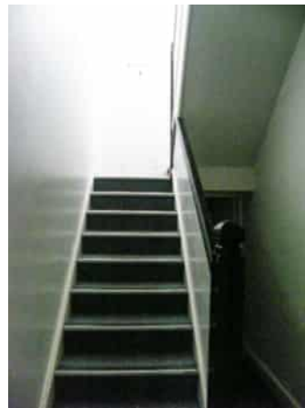
Photo 34: Main stair, facing west
