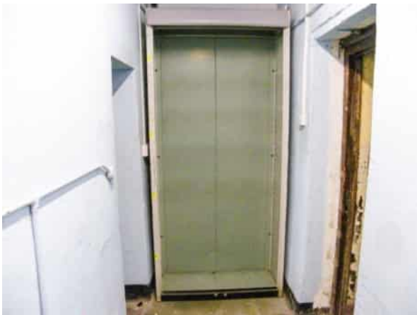
Photo 29: Corridor between cells, facing west (blocked by cabinet)
