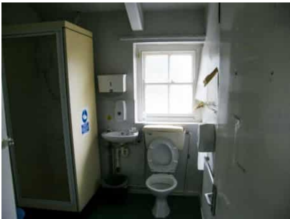
Photo 41: F2 bathroom, facing south
