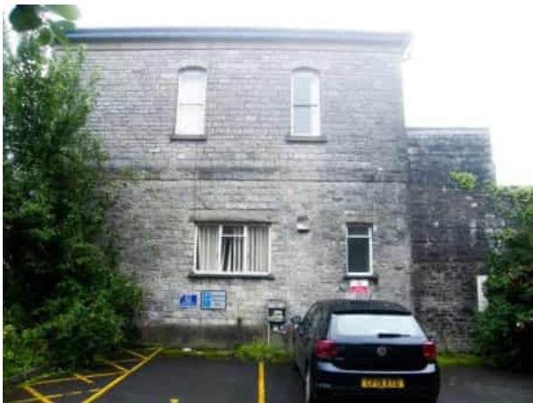
Photo 3: West elevation of Cowbridge Police Station
