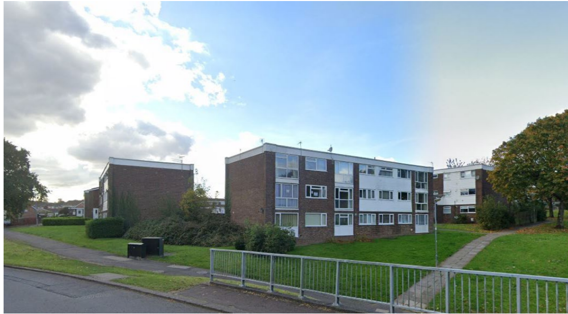
Glenwood, Circle Way West (immediate context); 3 storey, flat roof brick and render
