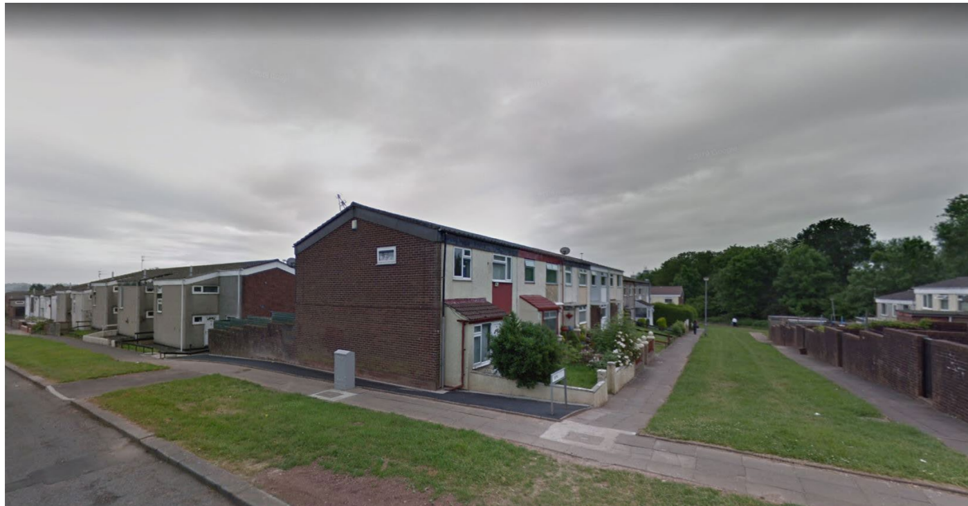
Brynfedw Estate (immediate context); A-symmetric roofs with gables on to Brynfedw road. Radburn layout with shared green space and rear parking courts
