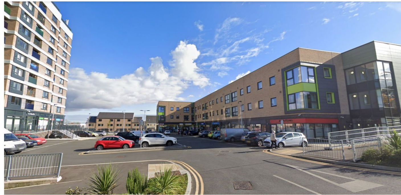
The Maelfa Centre; 3 to 10 storey contemporary flat roof commercial and residential development in brick and cladding, with 2/3 storey housing with pitched roofs.
