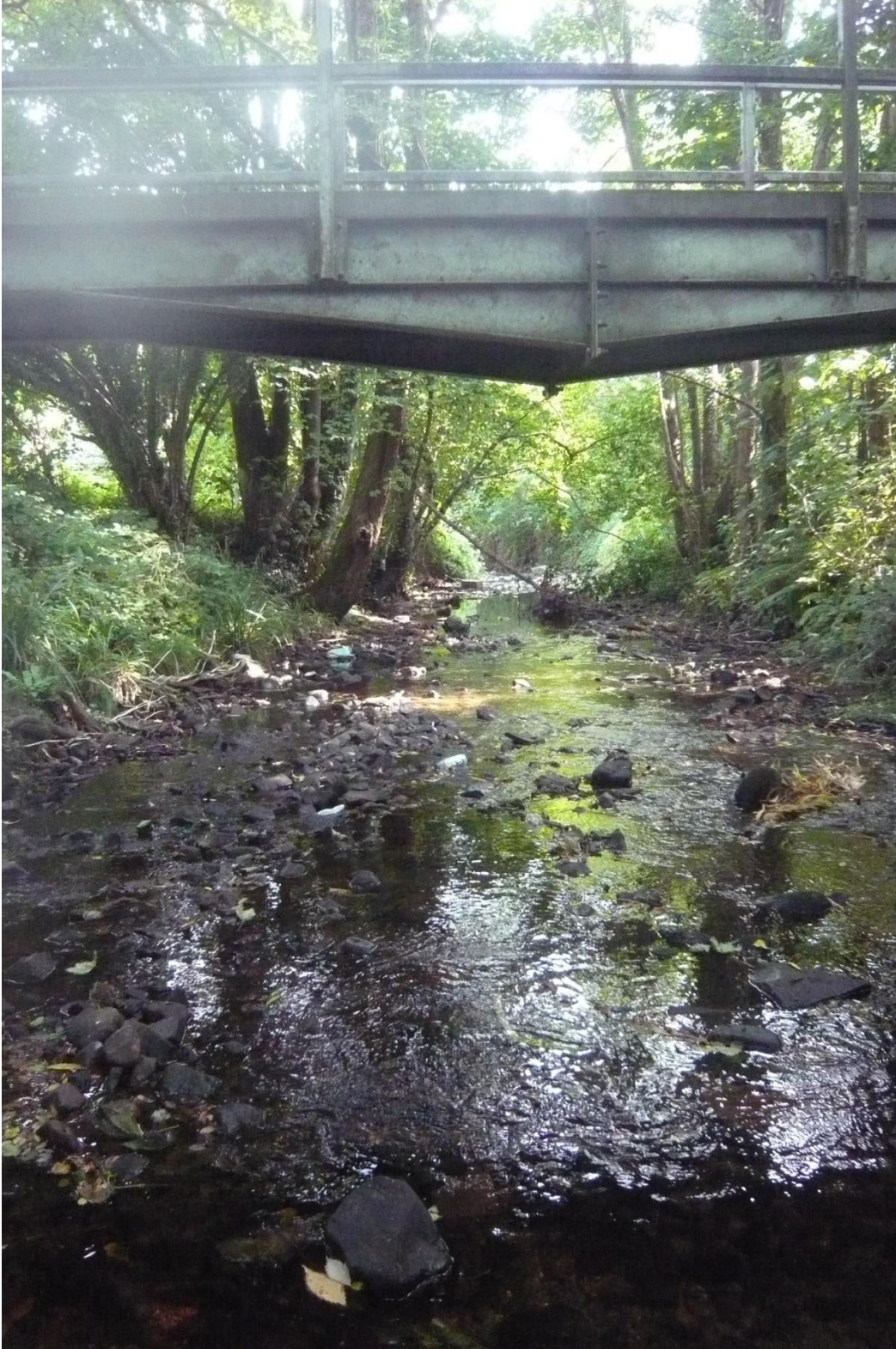
Photo 7: View from the upstream footbridge
