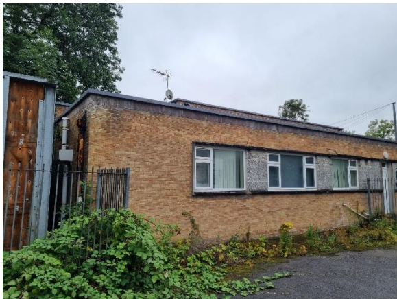
Figure 12 - The northern aspect of Building B.
