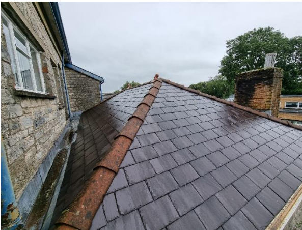
Figure 5 – Pitched roof on Building A.
