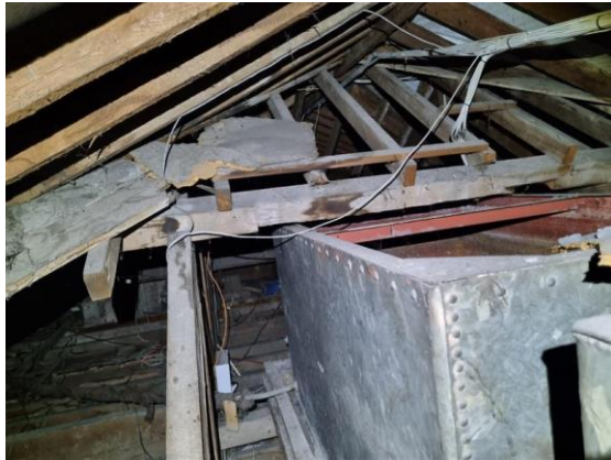
Figure 8 - Loft space in Building A.
