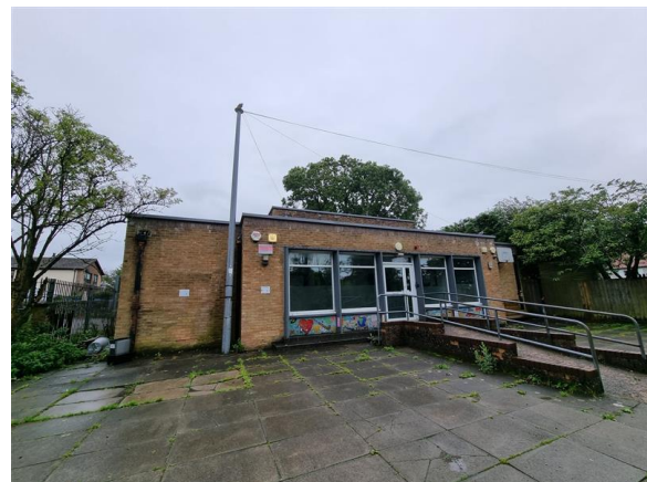
Figure 13 - The western aspect of Building B.
