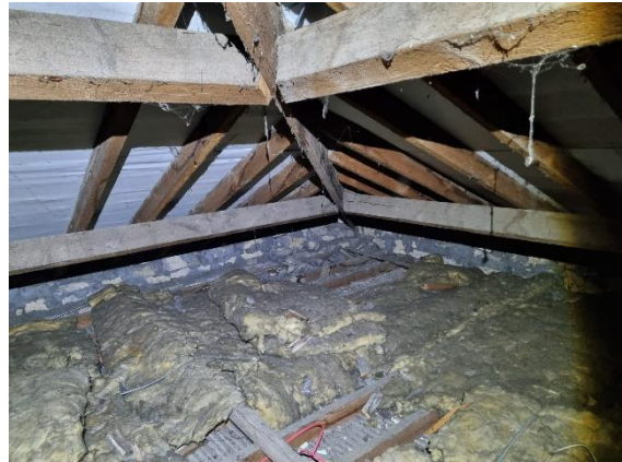
Figure 9 - Loft space in Building A.
